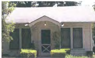
Appropriate wood window screens
