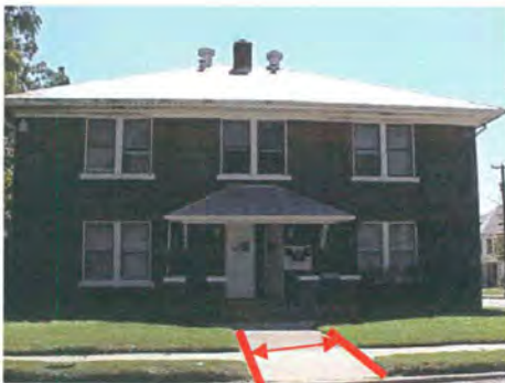
Typical example of front walkway on a residential property; Multi-family structures require a 4 foot walkway
