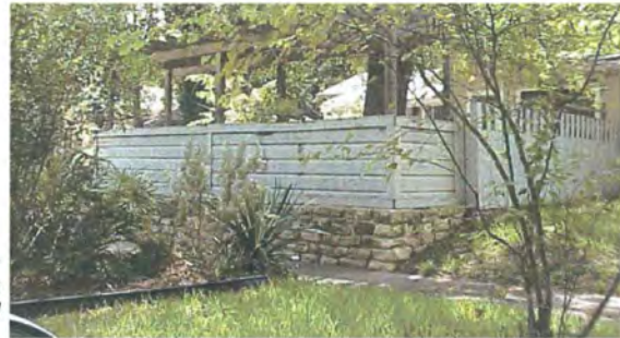
Examples of non-conforming fences in front yard
