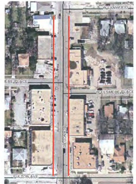
Aerial view of Blanco Road, depicting the shallow setbacks, and head-in / rear parking configuration.
