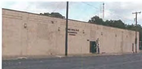
Non-conforming example of a commercial building with no window openings
