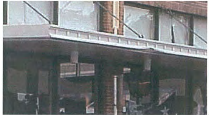
Example of commercial property with appropriately shielded exterior light fixtures
