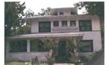
Typical two-and-a-half story residential structure
