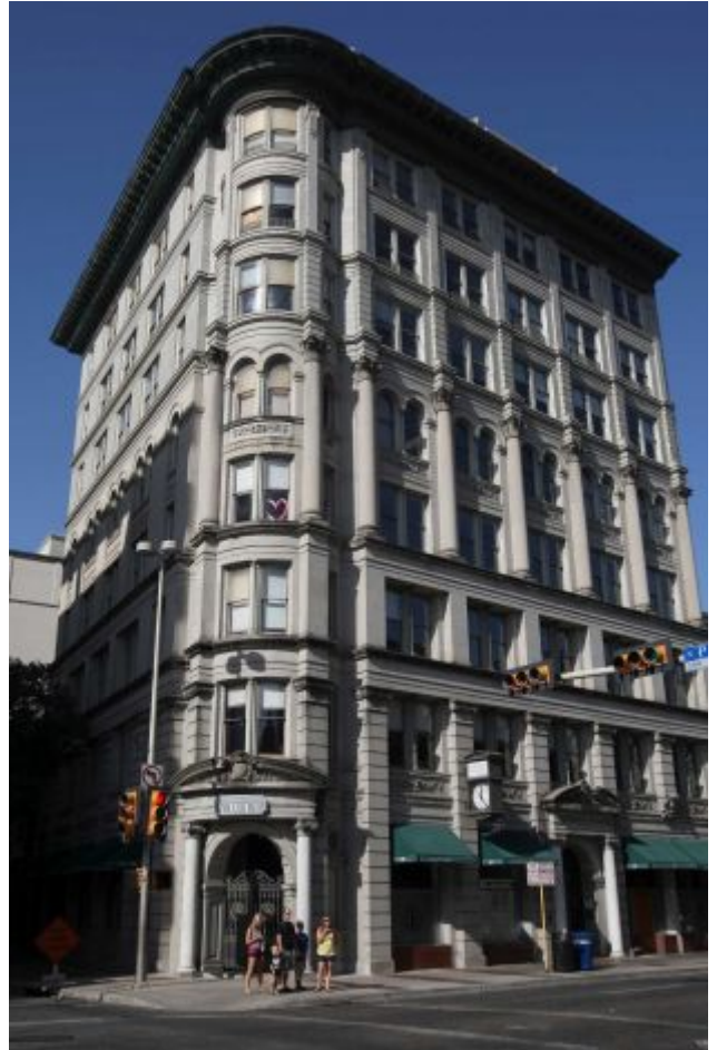
Fig 3.1 Corner Building on Commerce and South Presa
