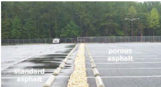
Fig 11.9 Pervious versus Impervious Surface Parking Lot
