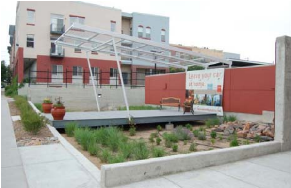
Fig 11.5 Storm water Control Landscaping Solution
