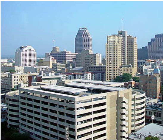
Fig 4.6 Parking Garage Without External Skin (Discouraged)
