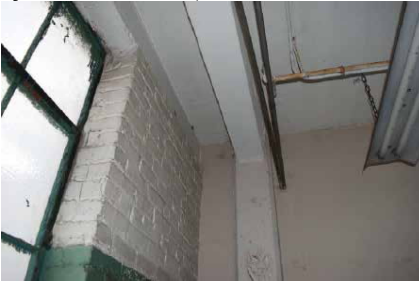
Figure 12 Typical framing of Clegg Building Brick wall separate from concrete encased steel beams and columns.
