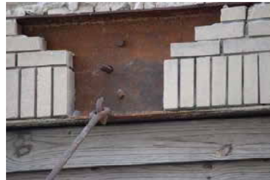
Figure 6 Damage to Brick and Canopy
