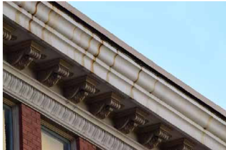
Figure 4 Staining on cornice Indication of moisture in framing
