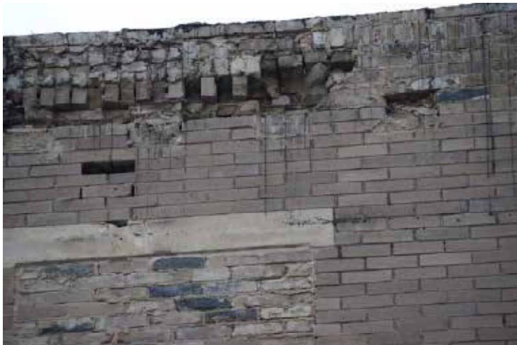
Figure 8 Damage to Face Brick
