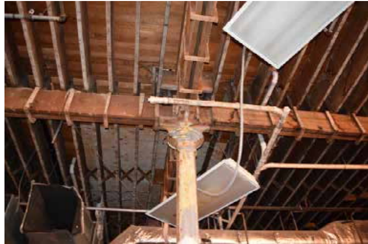
Figure 3 Typical Wood Floor Framing
