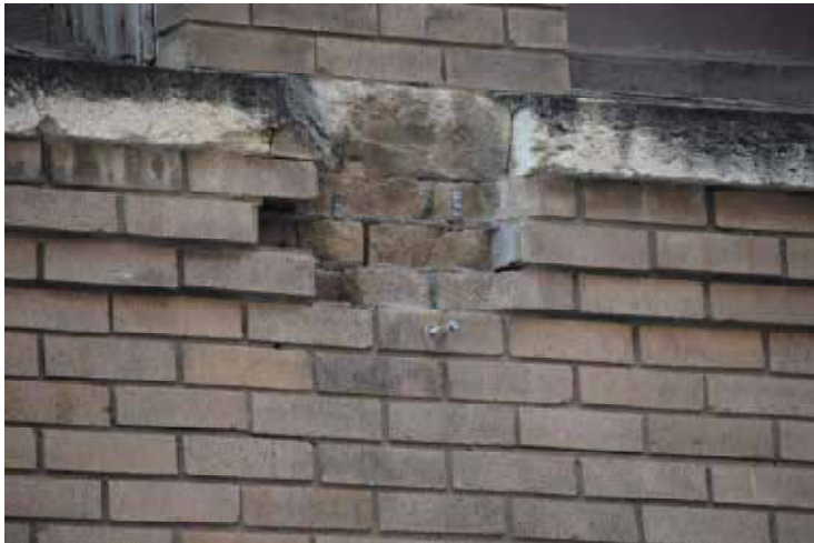
Figure 7 Damage to Face Brick
