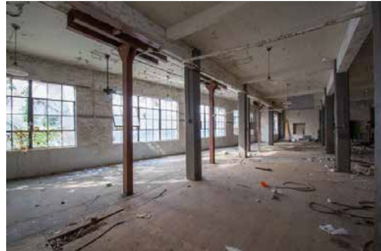
Figure 13 View of Framing inside of Clegg Building The existing framing with mix of column spacing, noting closely spaced columns And columns added during addition at river level.
