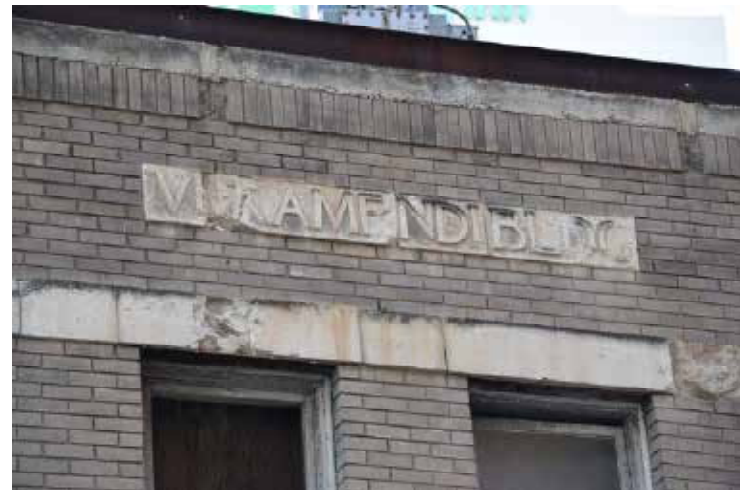
Figure 10 Detail of masonry damage
