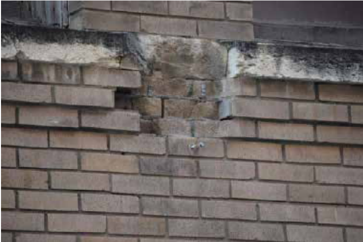
Figure 7 Damage to Face Brick
