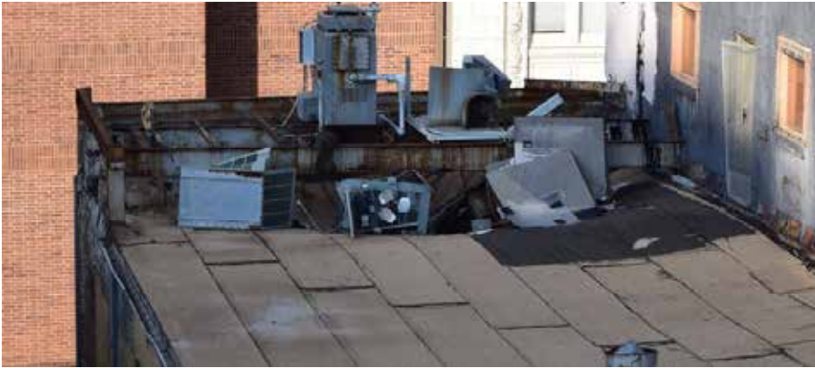
Figure 11 Failure of Roof behind Façade
