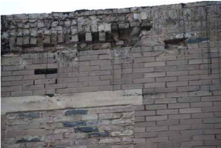
Figure 8 Damage to Face Brick
