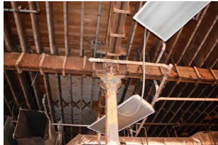
Figure 3 Typical Wood Floor Framing
