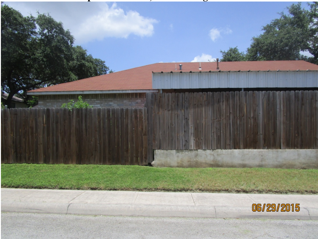
Fence built atop concrete slab, measures eight and a half feet tall
