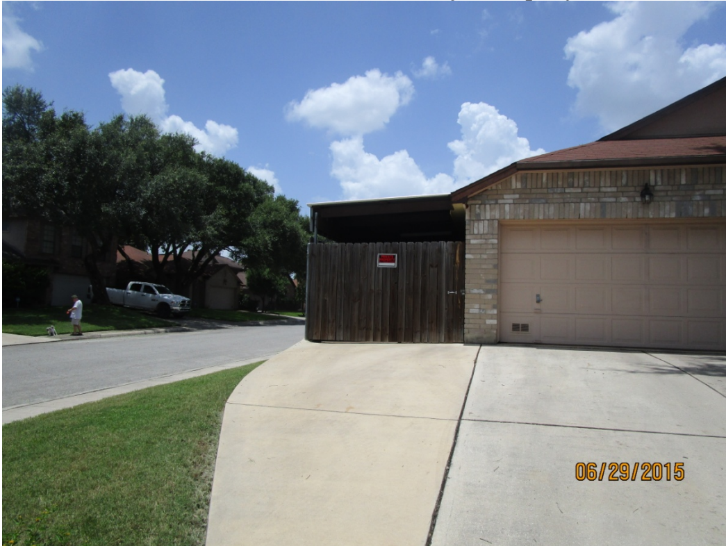
Fence built atop concrete slab, measures eight and a half feet tall
