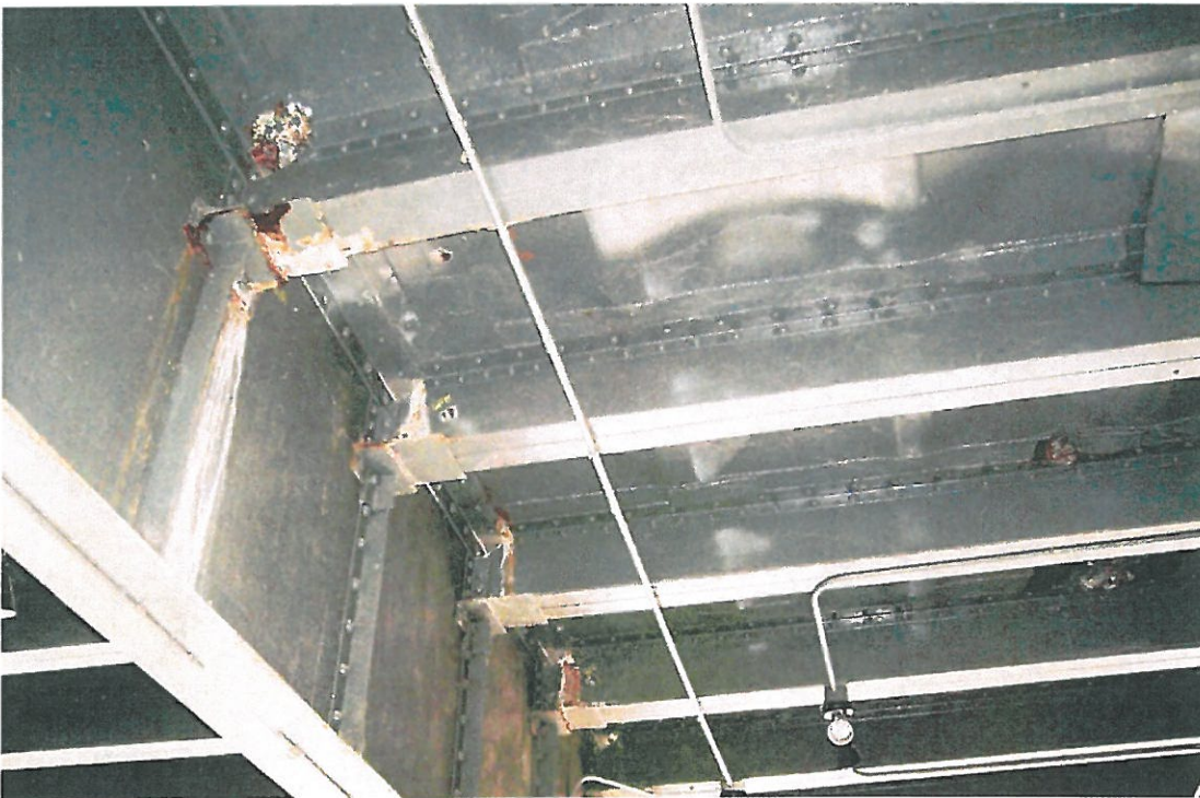
Figure 8: Underside of Crockett Bridge (Floor Beam and Stringers with corroded connections)
