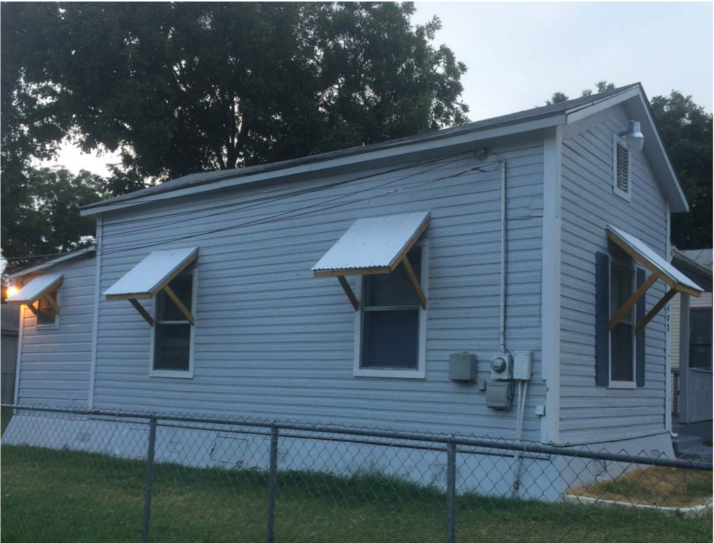
new corrugated metal window awnings - 403 burleson
