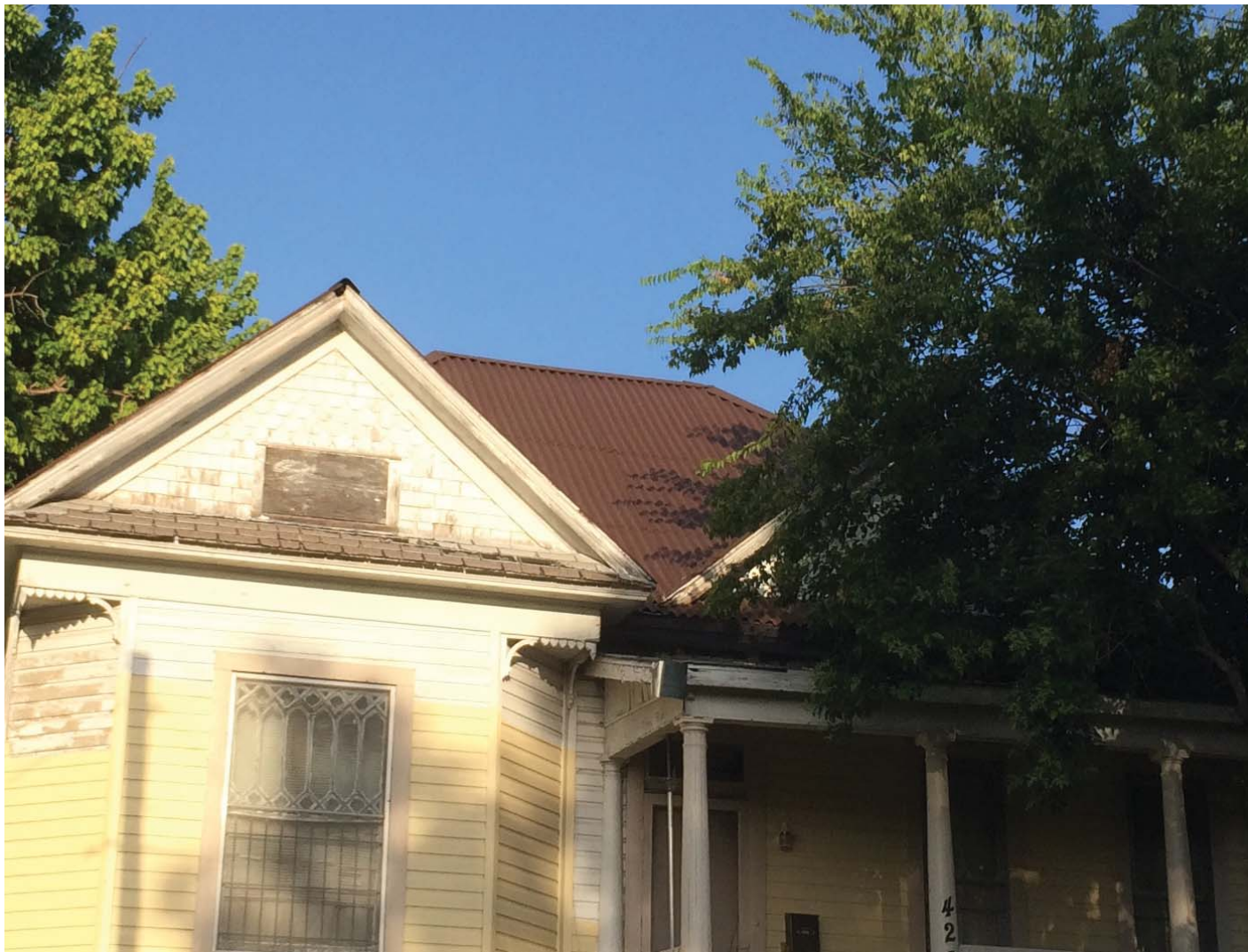
new corten corrugated metal roof - pine street
