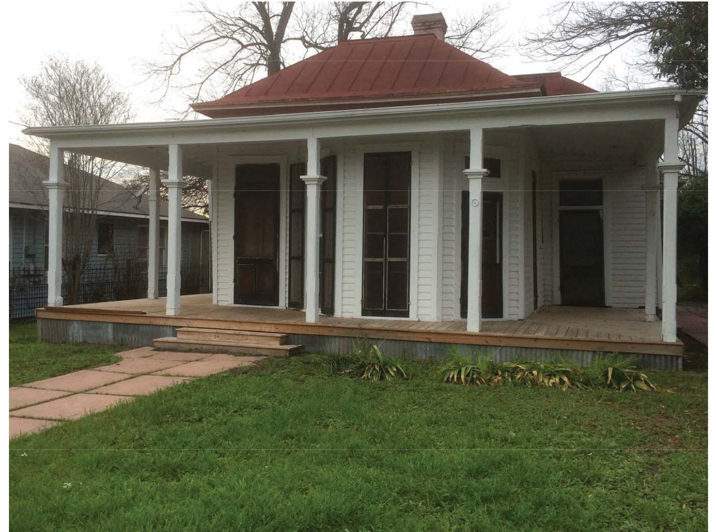
corrugated metal foundation skirt, weathered metal roof - lamar street
