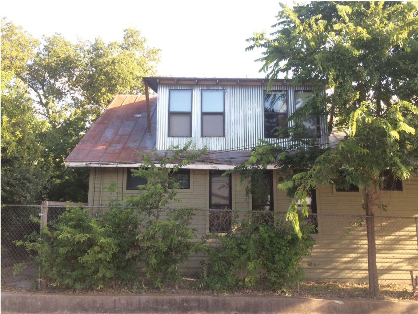
corrugated metal siding , weathered metal roof - 712 n. mesquite
