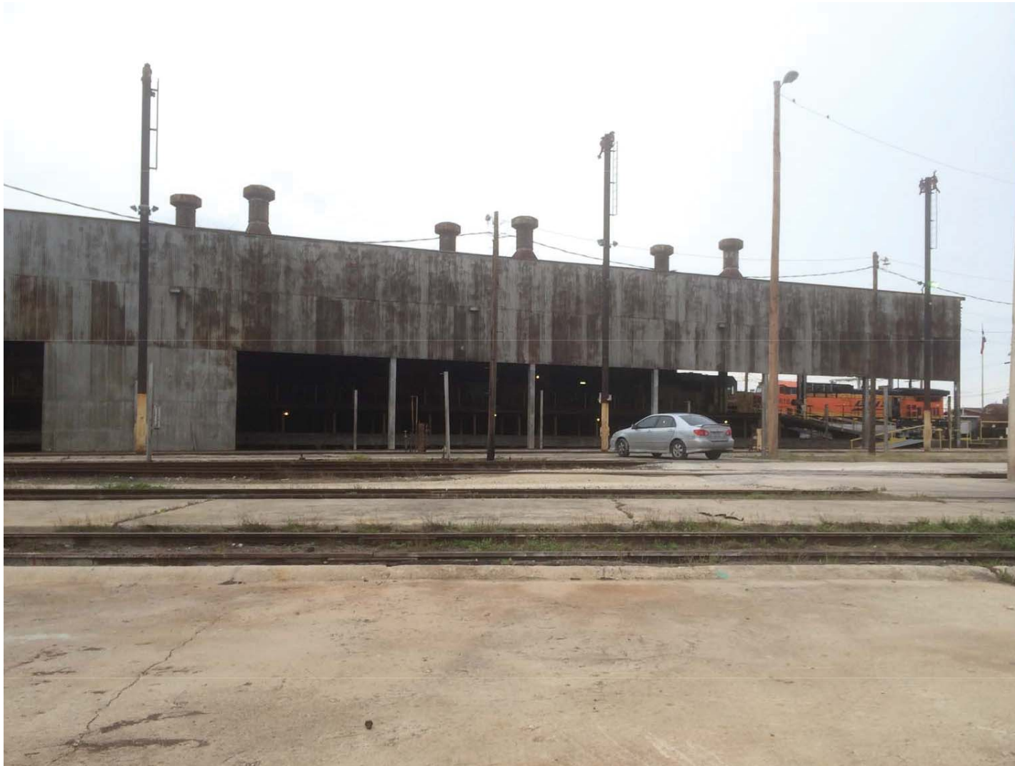
north edge of neighborhood - railyard buildings - weathered galvanized corrugated siding
