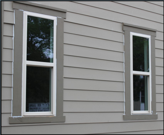
Vinyl windows installed with nailing strips cannot be masked by wood trim and do not provide an option for wood screens set within the trim.
