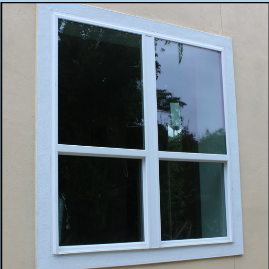
Vinyl windows with a flush flange or nailing strip protrude beyond the window trim and are not recommended.
