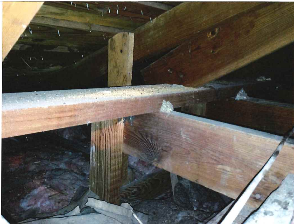
2" X 6" ceiling joists and 2" X 6" top plates were not used over the 1957 addition. The original cornice boxes were left in place, making the height of the ceiling in the second floor room equal to the height of the soffits. The photograph shows the top plate along the original north wall of what was the east end sleeping porch. Looking north past the top plate is the original cornice box which was, in essence, roofed over.
