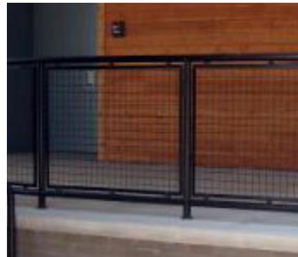
FENCE TYPE 1 DESCRIPTION: STEEL ANGLED WITH 2X2 METAL MESH WELDED TOGETHER PAINTED: PT-4 (ACCESS GATES SIMILAR)
