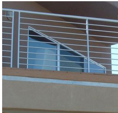
RAILING TYPE 1 (BALCONY) DESCRIPTION: 2X2 STEEL POSTS WITH HORIZONTAL PICKETS WELDED TOGETHER PAINTED: TO MATCH BALCONY COLOR
