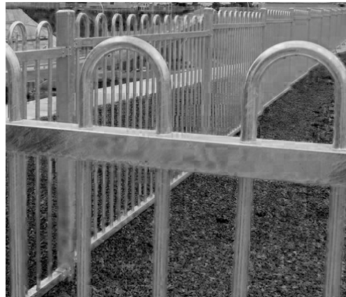
FENCE TYPE 3 DESCRIPTION: 2X2 STEEL POSTS WITH DECORATIVE LOOP PICKET FENCE WELDED TOGETHER PAINTED: PT-7 (ACCESS GATES TO MATCH)
