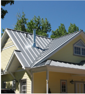
STANDING SEAM METAL ROOF COLOR: GALVALUM
