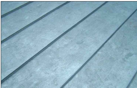
STANDING SEAM METAL ROOF TO MATCH EXISTING
