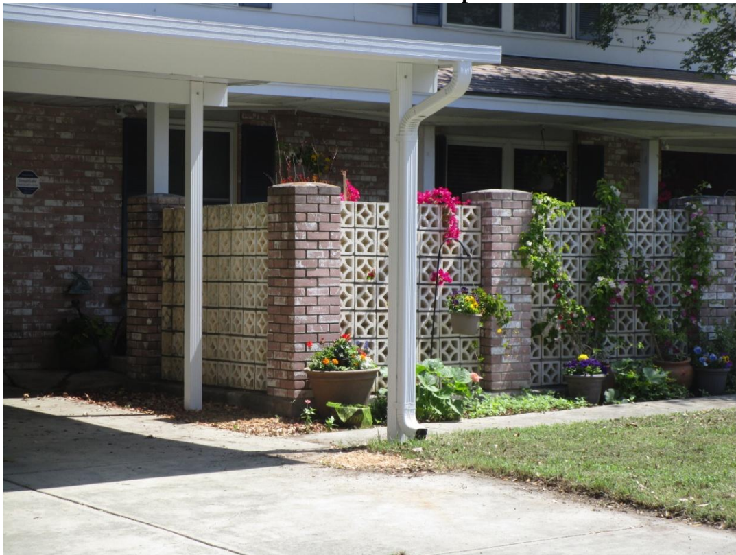
Gutters installed on carport
