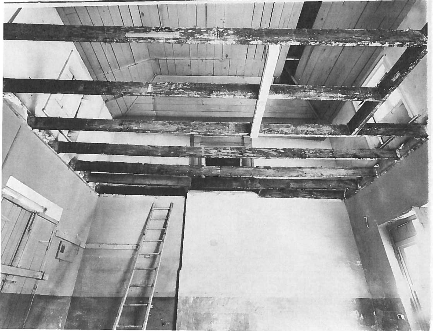
Figure 15. Interior of the Navarro Store and Office, looking up through charred second-floor joists, ca. 1962.
