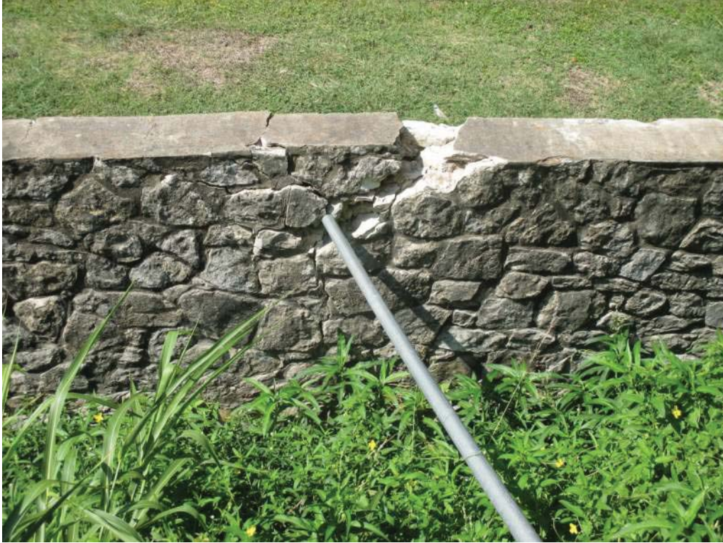
Photo 5: Failed section of north drainage channel wall at a steel pipe brace.
