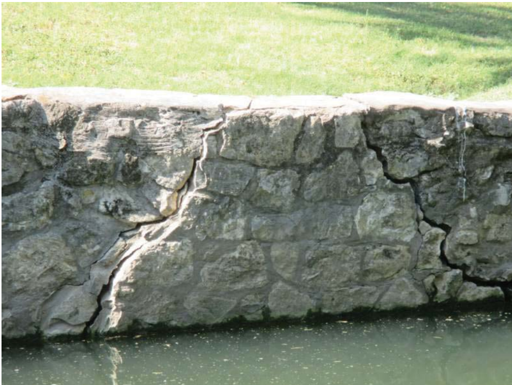
Photo 8: Segment of south drainage channel wall that has failed.
