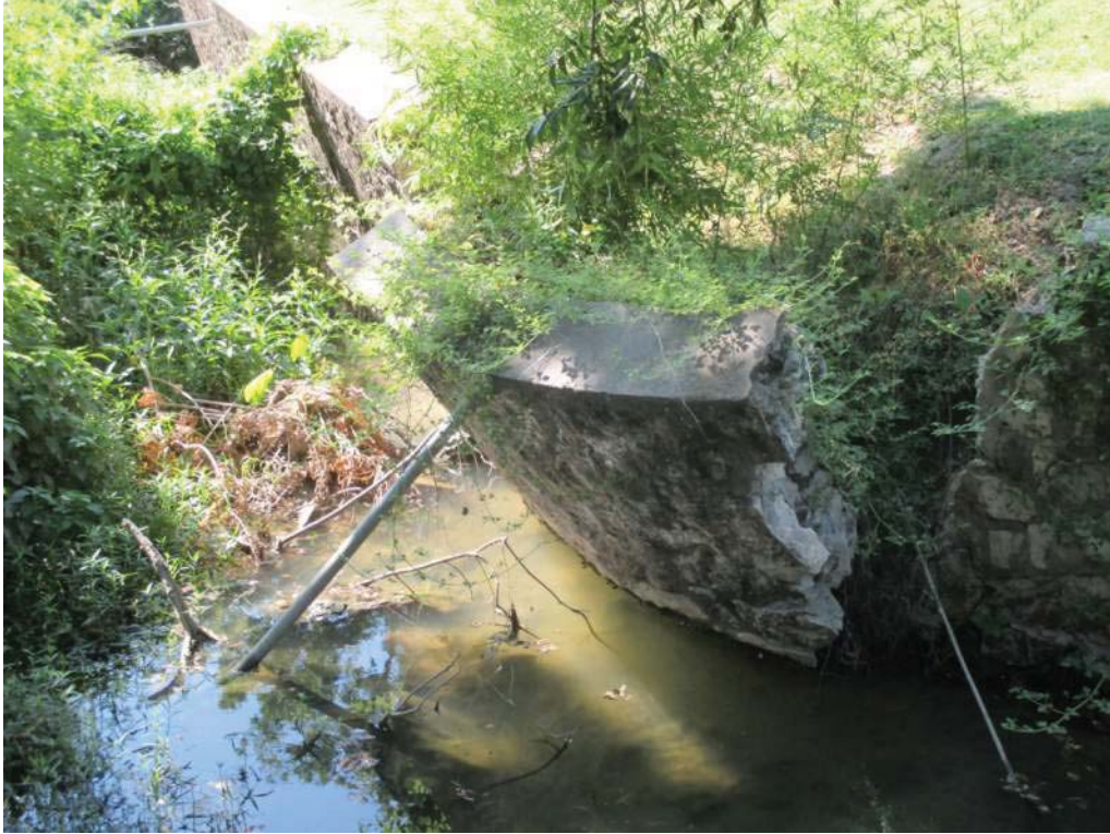
Photo 9: Collapsed section of south drainage channel wall.
