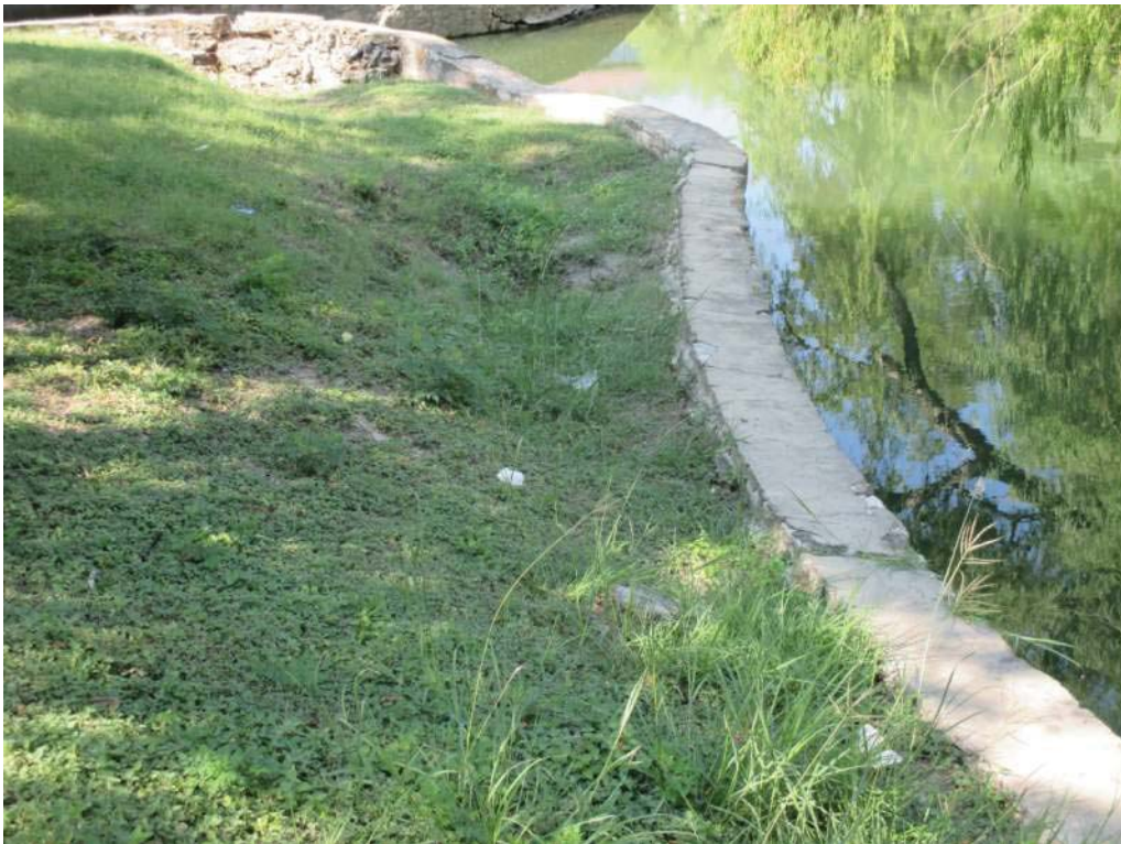
Photo 4: Top of north wall at the San Antonio River that has displaced and allowed soil behind wall to subside.
