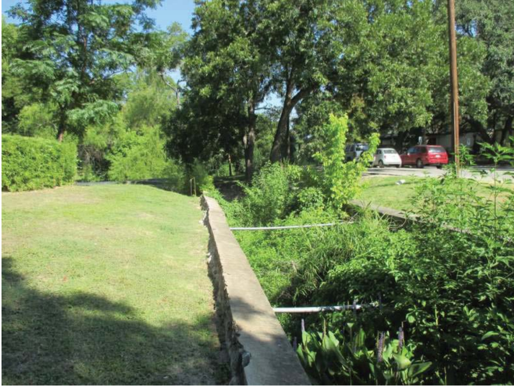
Photo 11: Drainage channel walls leaning at top looking west.
