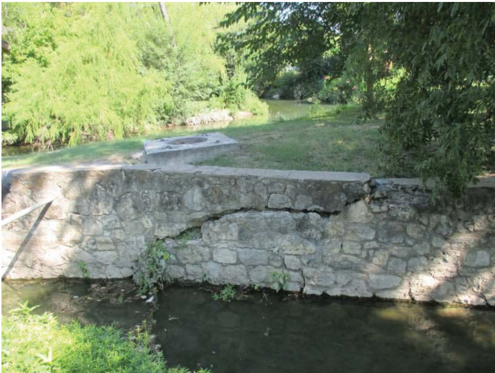
Photo 6: Severely cracked and failed section of north drainage channel wall.
