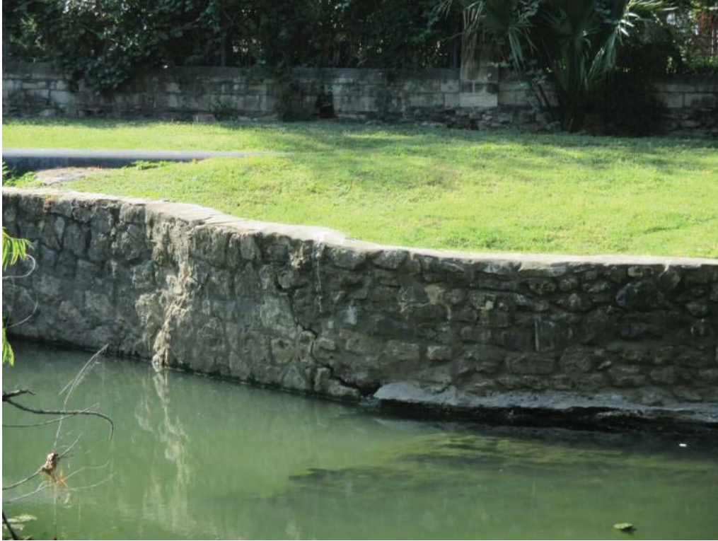
Photo 7: Cracked and failed section of south drainage channel wall.
