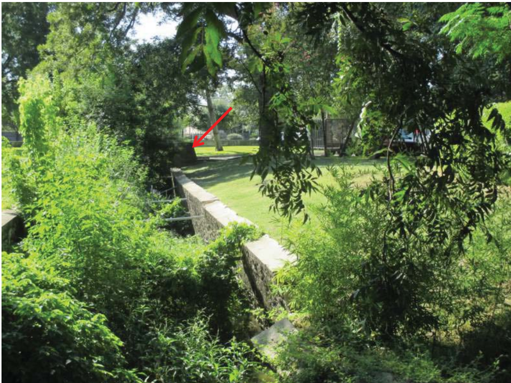
Photo 10: Drainage channel walls leaning inward and braced with steel pipe, looking east. The existing bridge abutment at Curiosity Lane is visible at arrow.
