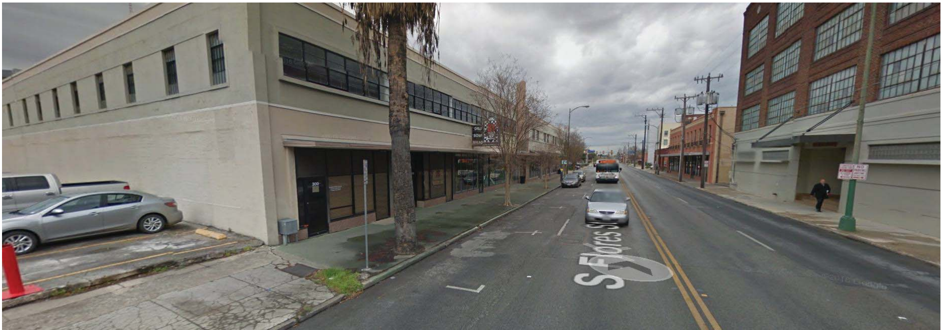
View of Subject Property from S. Flores St. (looking southeast from the west side of the property)
