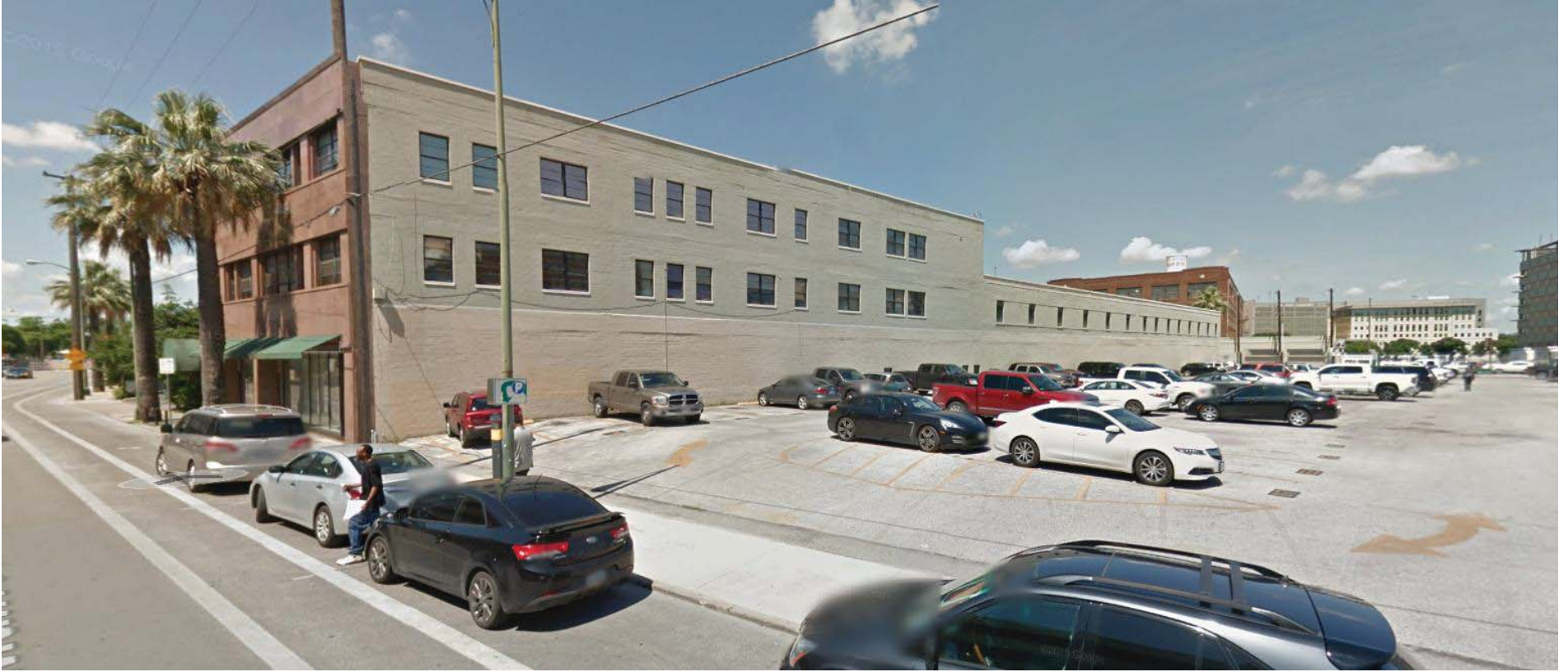
View of Subject Property from S. Main Ave. (looking southwest from the east side of the property)
