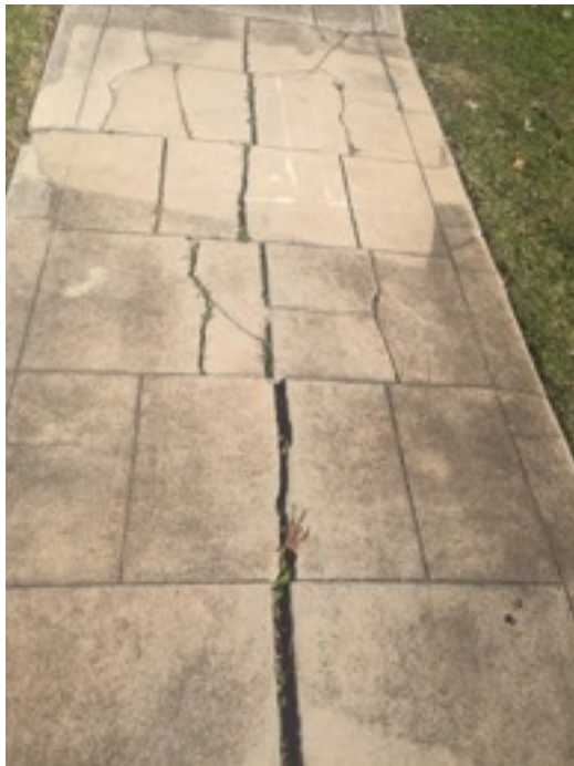
Broken Sidewalks at Commanders House.
