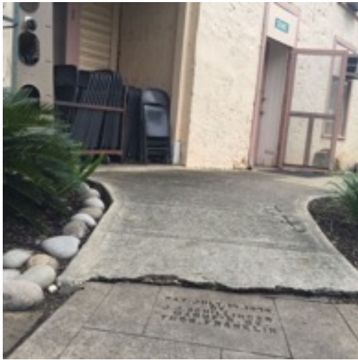
Broken Sidewalks at Commanders House.
