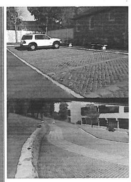
**float up over time**. It allows grass to grow up thru the surface; turfstone can be completely invisible if covered with sod while creating a long lasting reinforcement system for grassy areas.
