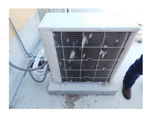
AC units will need to be either combed out or replaced.
