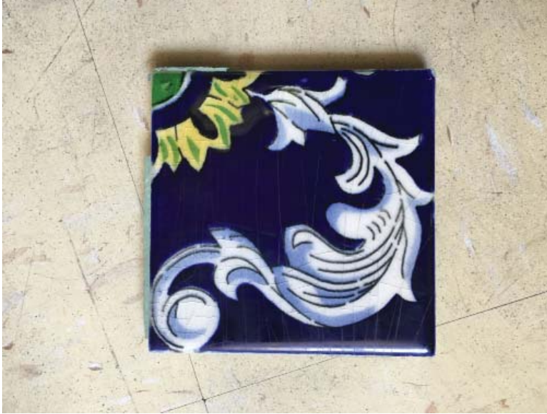
EXISTING TILE ON NORTH AND EAST FACADE 4 1/4" X 4 1/4"
