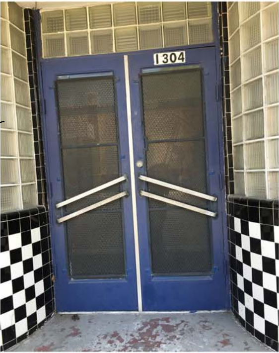
103 - DOOR IS UNDERSIZED FOR EMERGENCY EGRESS
