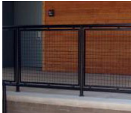
BALCONY RAILING DESCRIPTION: STEEL ANGLED WITH 2X2 METAL MESH WELDED TOGETHER PAINTED: PT-2 (ACCESS GATES SIMILAR)
