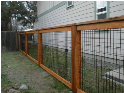
FENCE TYPE 1 DESCRIPTION: WOOD FRAME WITH METAL MESH PAINTED: TBD (ACCESS GATES SIMILAR)
