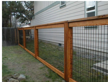
FENCE TYPE 1 DESCRIPTION: WOOD FRAME WITH METAL MESH PAINTED: TBD (ACCESS GATES SIMILAR)
