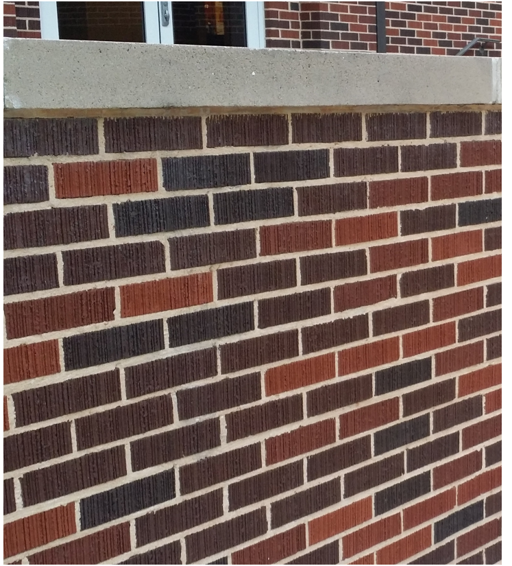
07 20 IN. HEIGHT BRICK SEAT WALL -CMU CONSTRUCTION WITH CAST STONE CAP AND BRICK TO MATCH EXISTING
