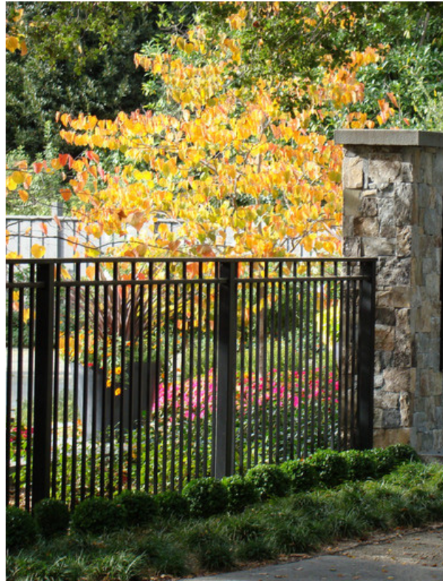
05 7 FT 6 IN DARK BRONZE FENCE WITH 8 FT CUT LIMESTONE COLUMNS
