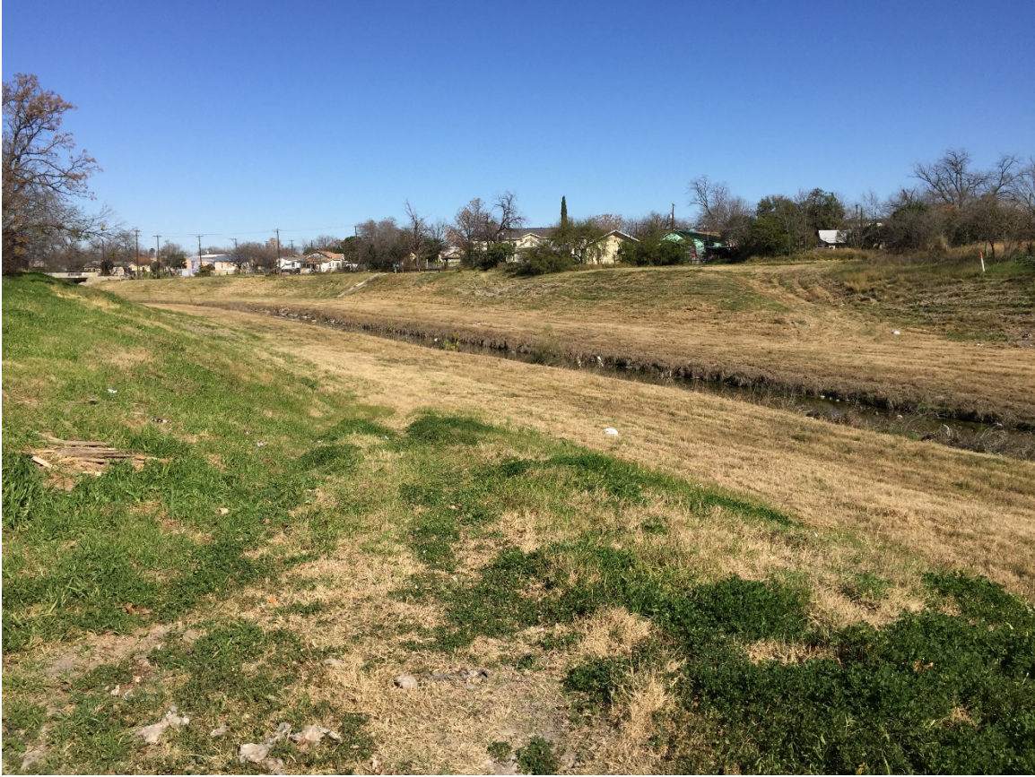
Figure 2 Alazan Creek Looking Downstream
