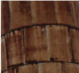
2. Existing weathered metal retained. Clear coat finish over patina.
