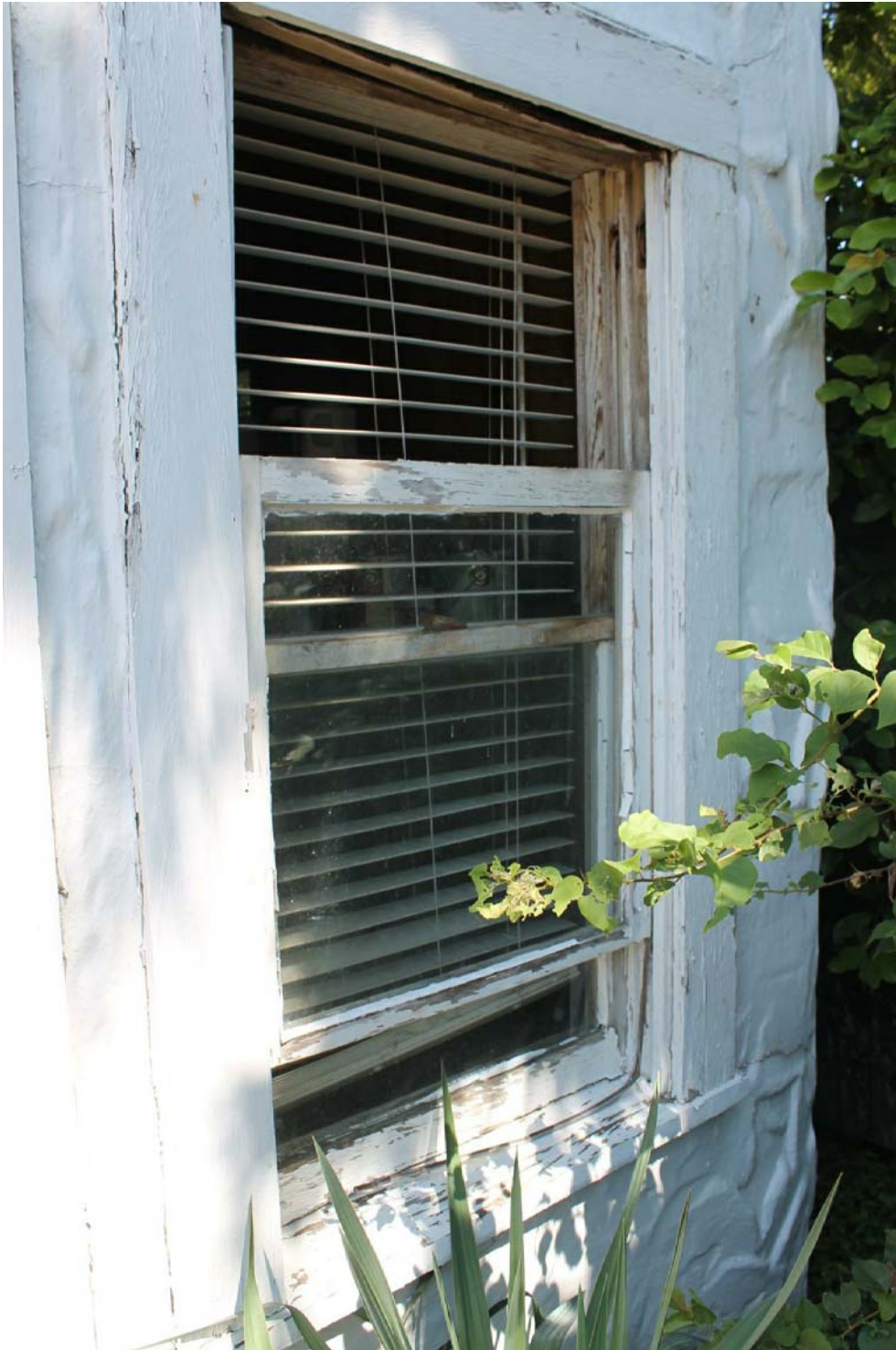
Detached garage storage room window and rotten trim
