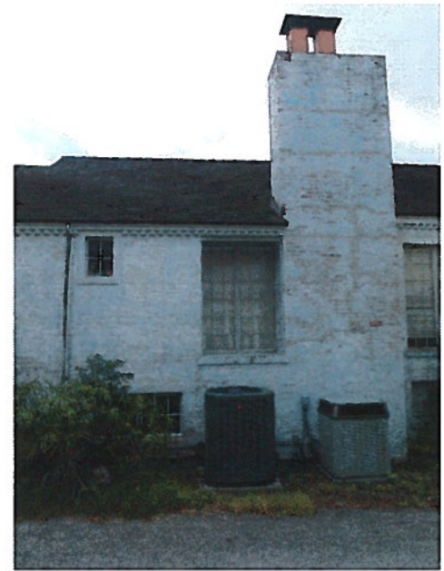
Detail of repointed masonry joints, replaced broken/cracked masonry (at window jamb/head corner), new painted redwood eave trim and copper drip edge (typical at all roof locations)
