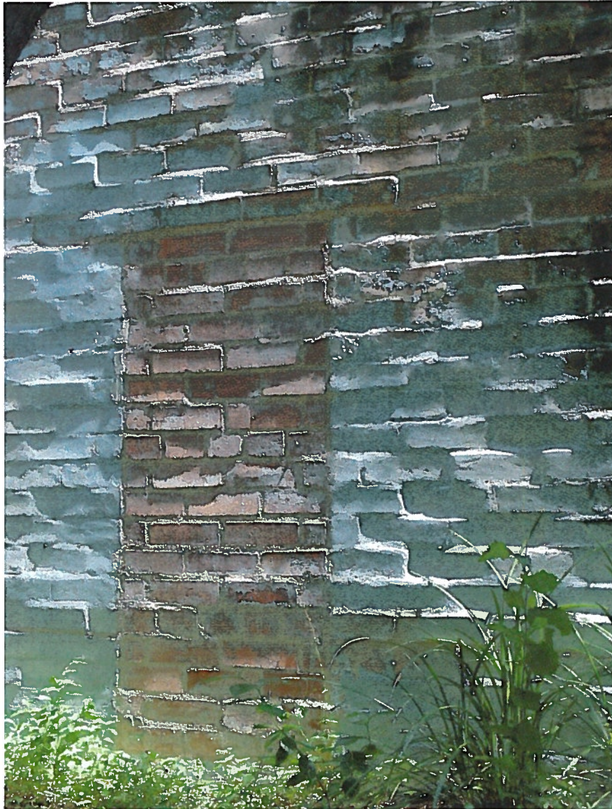
Street Façade – (left) Detail of infill masonry below stairs – tried to emulate slightly irregular placement of individual bricks seen in existing masonry; (right) Detail of repointed masonry joints using white masonry cement, and medium coarse sand in 1:3 ratio similar to existing mortar (picture taken below cantilevered second floor kitchen next to garage door)
