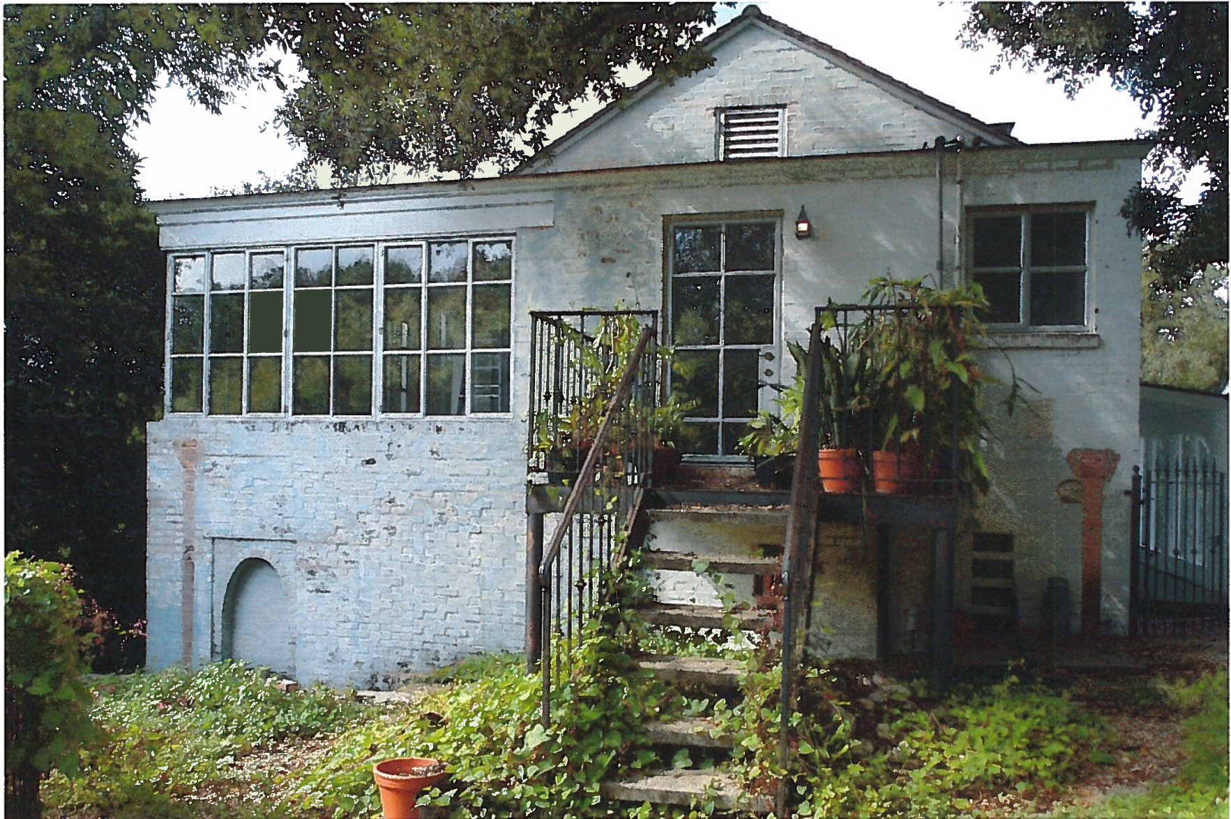
Rear Façade (Northeast Elevation) – New roof beam and trim and casement windows at second floor sunporch (upper left) to replace those damaged by fire; new glazed rear door and upper right window to match replacement windows at sunporch; new perimeter eave trim and copper flashing throughout; new roofing over new tapered roof insulation at flat roof area; new attic louver/access door in gable to replace existing damaged by fire department; repointed masonry joints in numerous locations; new decorative masonry "lattice" over first floor window (partially obscured by metal stairway – detail later). Note: circular hole in masonry on lower far right will be filled by first floor kitchen exhaust hood once interior renovation begins.
