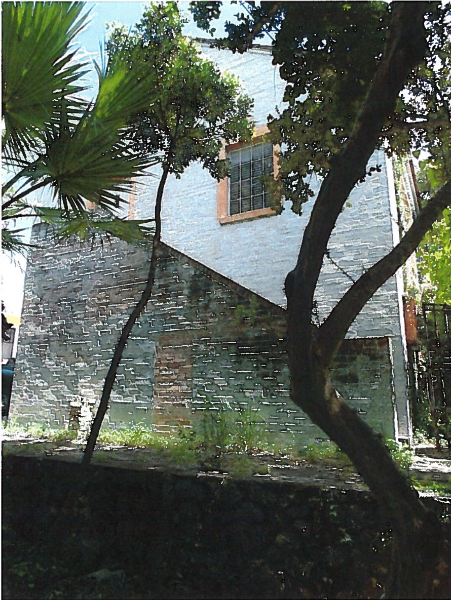
Street Façade (Southwest Elevation) – repointed masonry in various places; infilled access door below stairs with D'Hanis solid bricks (one of a variety of bricks used in original construction); re-installed existing Ludowici roof tiles over new underlayment with copper flashing and new redwood eave trim to match existing profile and dimension throughout (existing trim had significant wood rot and termite damage); new board and batten siding (dimensions and profiles matching existing) on cantilevered second floor kitchen over garage below (existing siding had significant wood rot); refurbished and repainted existing front door.
