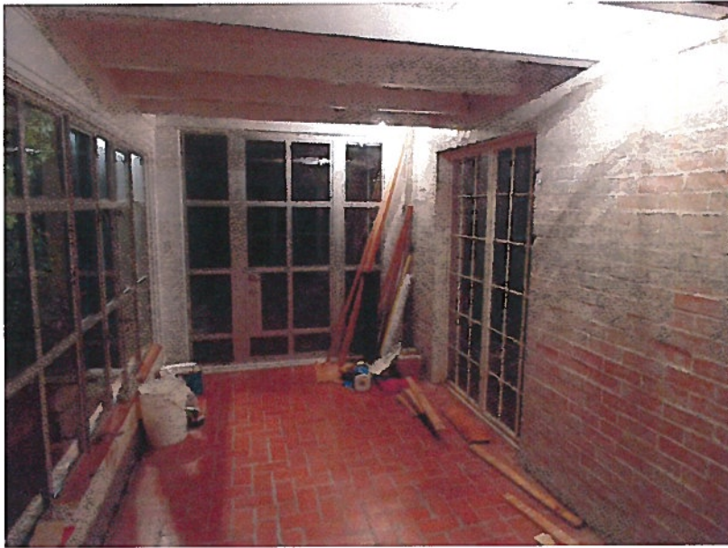
Interior of sunporch (repair of fire damage): replacement windows on left and new glazed door with sidelites at center (access onto existing balcony); last two bays have replacement ceiling decking (destroyed by fire); new lighting (reinstallation of fixtures already in my possession)
