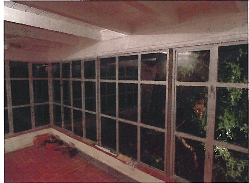
Replacement windows, new wood roof beam above windows with finish trim; existing roof beams and decking repainted; existing tile floor cleaned
