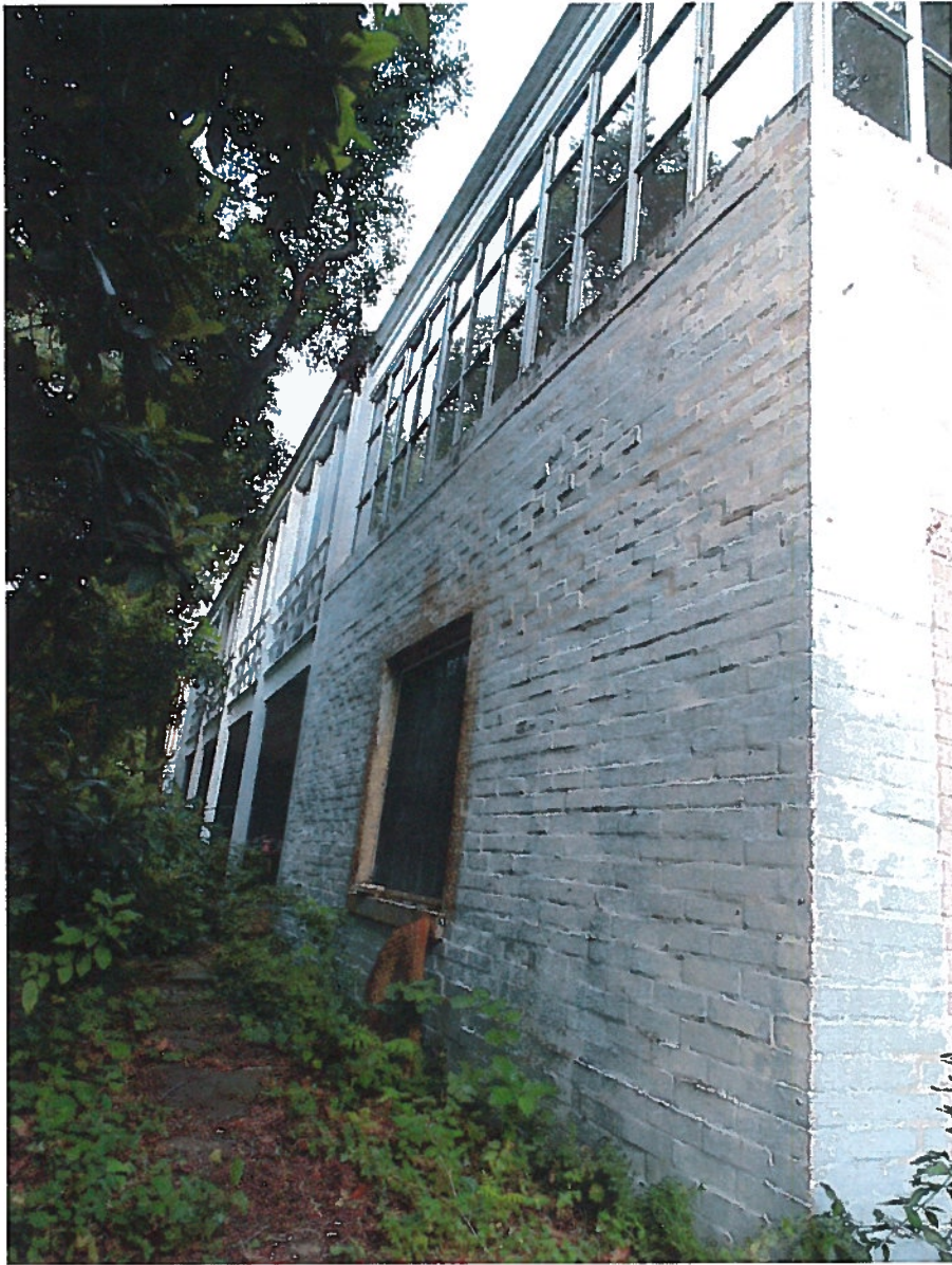
Side Façade (Southeast Elevation) – Repointed masonry throughout; new roof beam/trim and windows at second floor sunporch; replacement 6x6 wood porch columns, new balcony porch flooring, railings and screening
