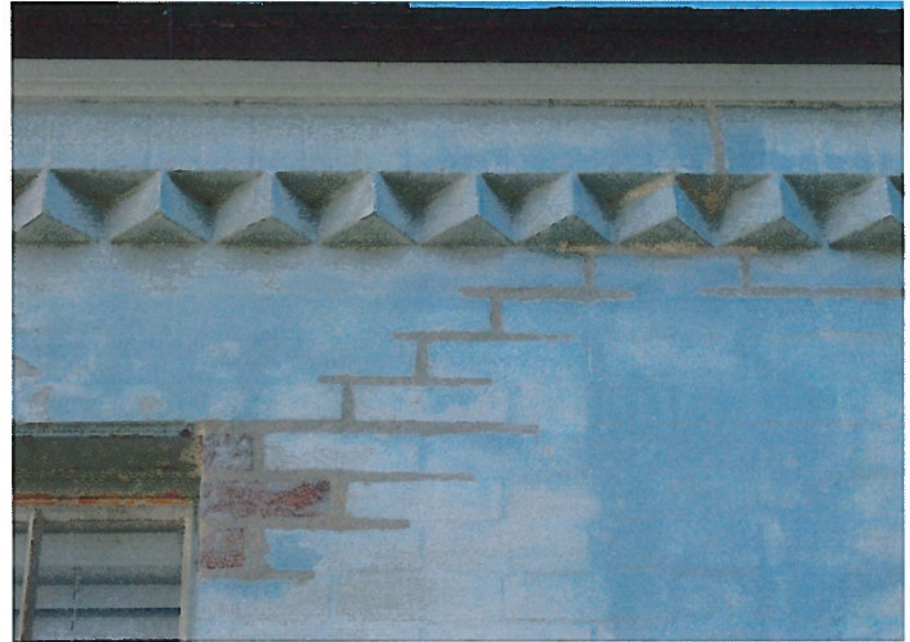
Detail of repointed masonry joints, replaced broken/cracked masonry (at window jamb/head corner), new painted redwood eave trim and copper drip edge (typical at all roof locations)
