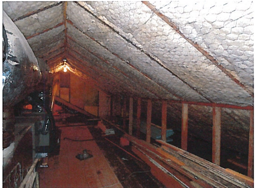
Attic showing new batt insulation at rafters with poultry netting support
