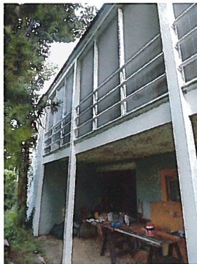
Side Façade (Southeast Elevation) – new porch columns; new porch flooring, railings and screening. Note: this elevation is difficult to photograph in its entirety due to tree canopies
