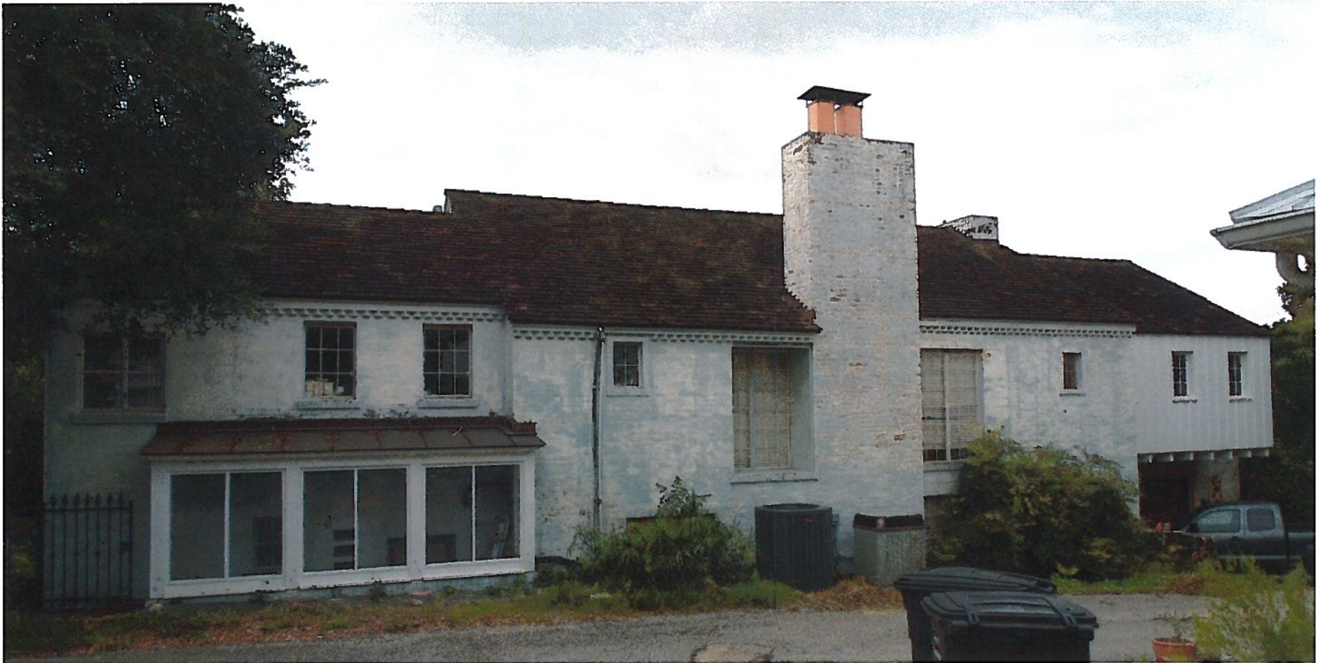
Driveway Façade (Northwest Elevation) – New replacement window far left upstairs to replace fire-damaged existing; refurbished roofing, copper flashing and perimeter eave trim as noted earlier (roof now has some hail damage – awaiting repair);repointed masonry in numerous locations; new standing seam copper roof over rear porch covering stairs down to first floor kitchen; also new glazed rain screen and wood frames at rear porch openings (to prevent flooding of stairwell – replaced existing “temporary” corrugated plastic panels); new outdoor HVAC condensing unit (taller one on left) relocated from former location near garage; new board and batten siding, refurbished windows and insulated floor at second floor cantilevered kitchen (far right of photo)
