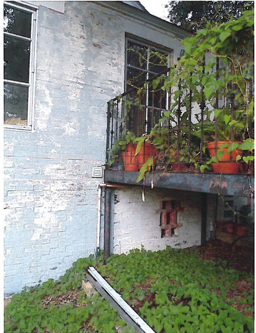
Detail of replacement glazed door above and new brick "lattice" over first floor window (pattern of lattice confirmed by existing masonry evidence – original lattice was missing when residence was purchased in 1996, painting delayed until entire house can be painted)
