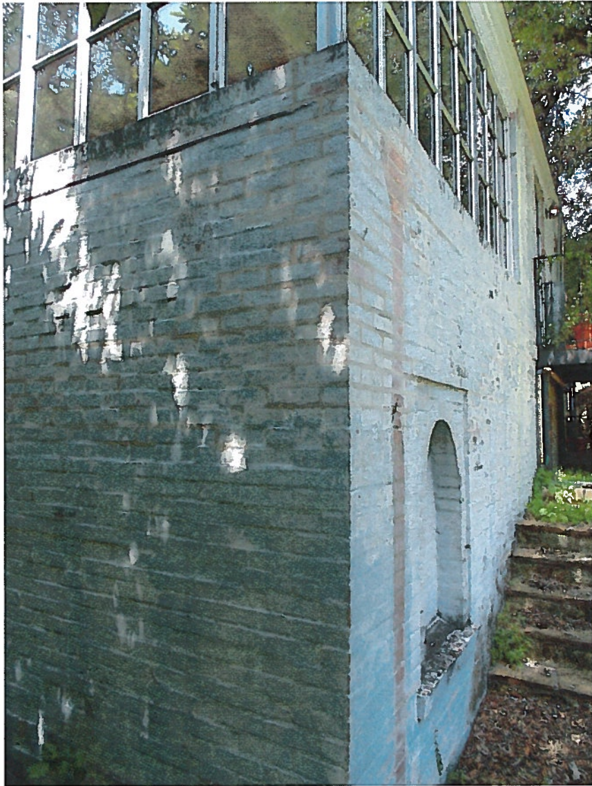
Detail of repointed masonry
