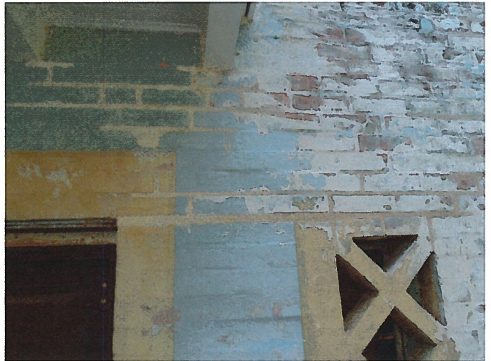
Street Façade – (left) Detail of infill masonry below stairs – tried to emulate slightly irregular placement of individual bricks seen in existing masonry; (right) Detail of repointed masonry joints using white masonry cement, and medium coarse sand in 1:3 ratio similar to existing mortar (picture taken below cantilevered second floor kitchen next to garage door)
