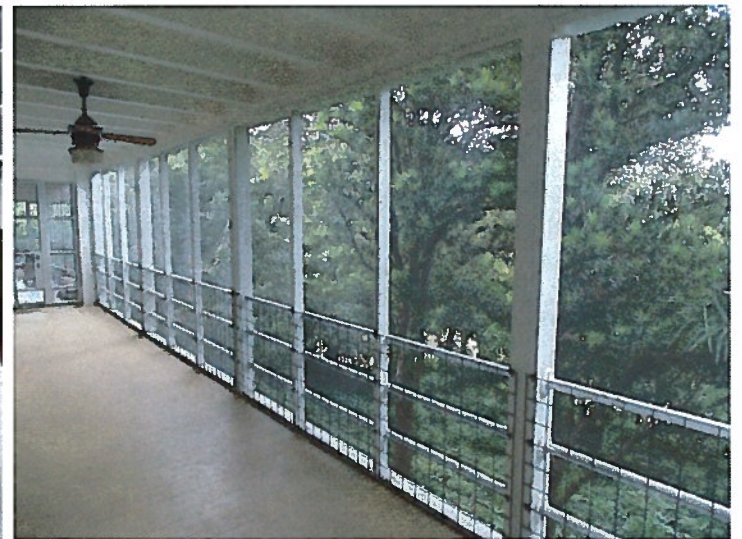
Side Façade (Southeast Elevation) – new porch columns; new porch flooring, railings and screening. Note: this elevation is difficult to photograph in its entirety due to tree canopies
