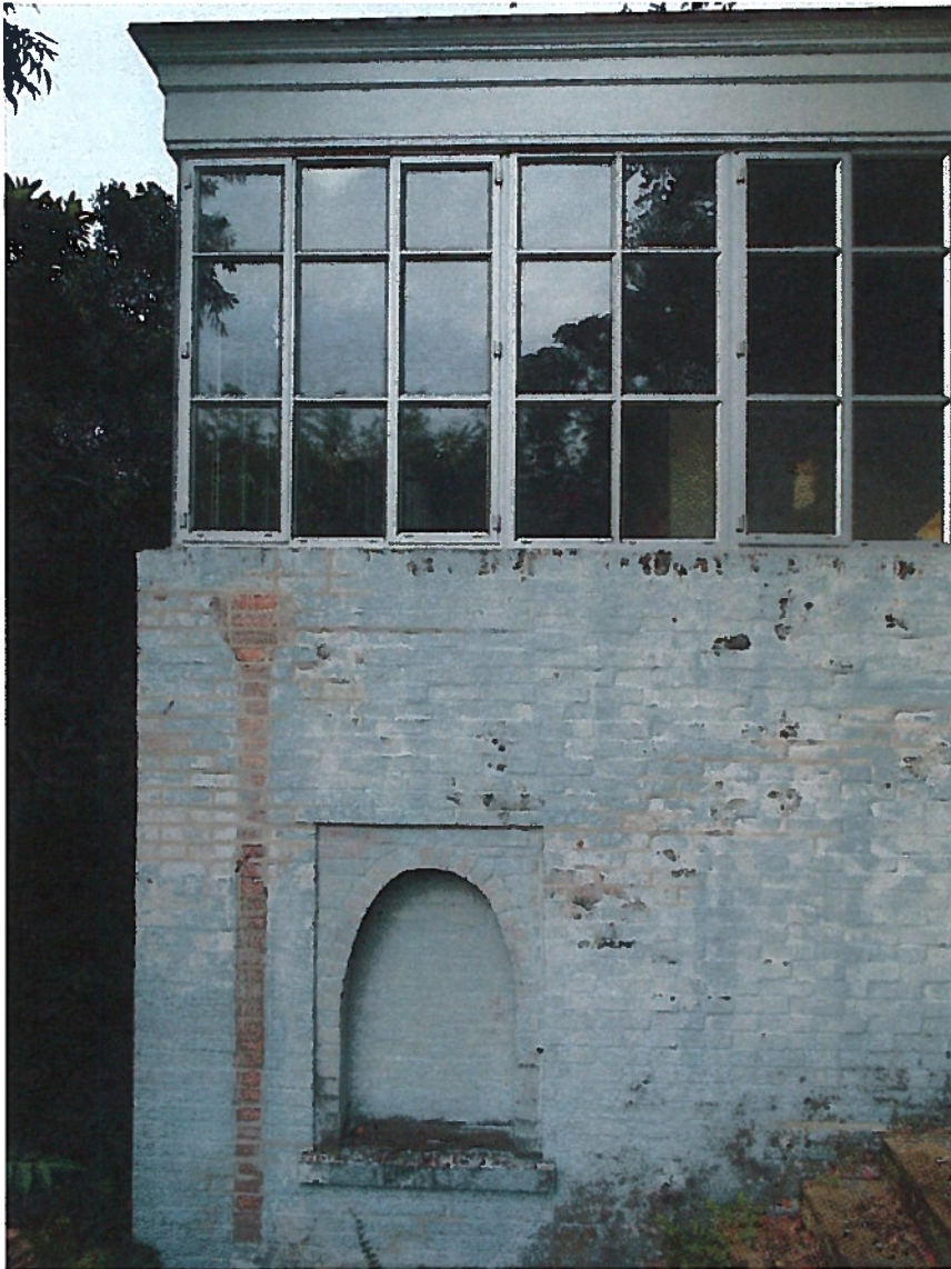
Detail of sunporch beam and replacement windows; repointed masonry, especially at exterior corner below windows. Note: former sheet metal downspout was damaged by roofing operations and removed – opening was infilled with D'Hanis solid brick
