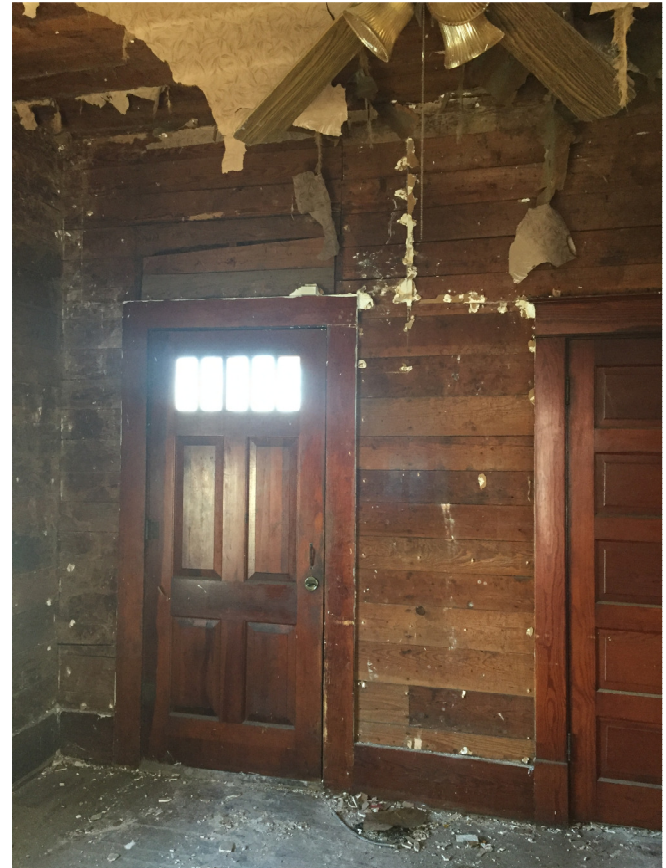
INTERIOR VIEW OF PORCH DOOR. A SEAM EXISTS ON THE RIGHT SIDE ABOVE THE DOOR BUT NO SEAM ON THE LEFT SIDE. NO EVIDENCE TO SHOW A PREVIOUS TALLER OPENING EXISTED. DOOR TRIM IS ALSO DIFFERENT FROM ORIGINAL TRIM.
