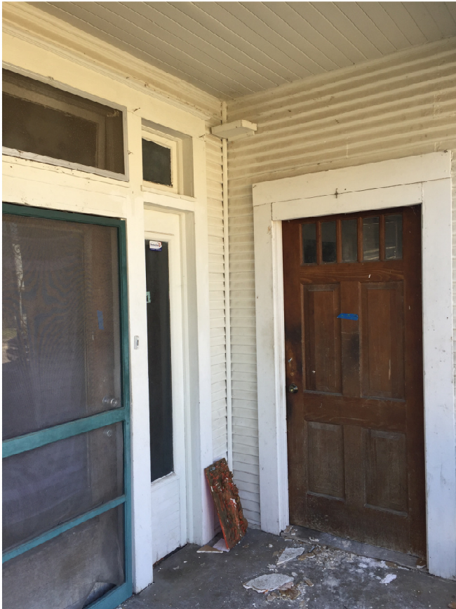
EXTERIOR VIEW OF PORCH DOOR. HEADER DOES NOT MATCH ADJACENT HISTORIC DOOR'S HEADER. ALSO NOTE THE SIDING ABOVE THE DOOR APPEARS INTACT AND THERE IS NO EVIDENCE TO SUGGEST A TALLER OPENING EXISTED THERE PREVIOUSLY. DOOR TRIM IS ALSO DIFFERENT FROM ORIGINAL TRIM.
