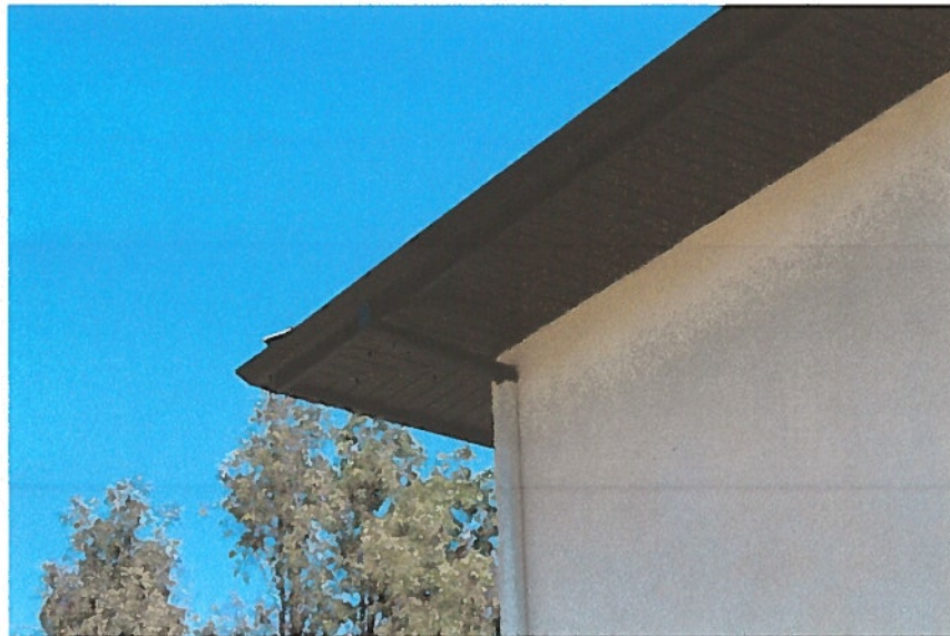
Temecula Ca. Soffit, Fascia, Gutters, Downspouts, Beam Cap, After Stucco
