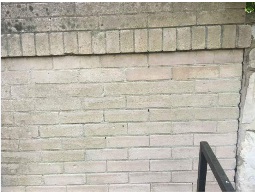
ELEVATED POOL BEAM FACED IN BRICK TO MATCH HOUSE
