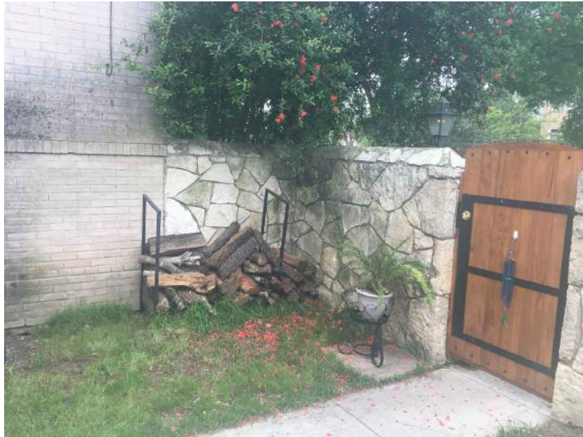
REPLACE EXISTING STONE WALL WITH NEW BRICK WALL TO MATCH EXISTING BRICK ON HOUSE
