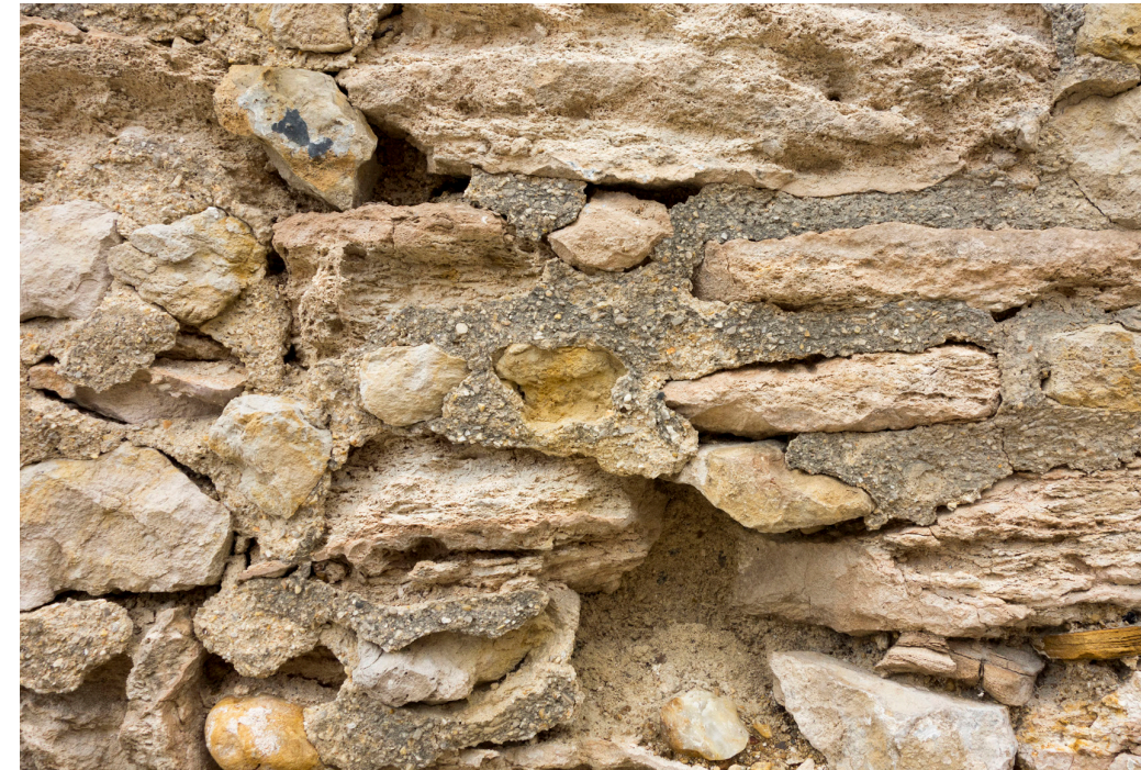
Severe material loss in the zone of rising damp.
