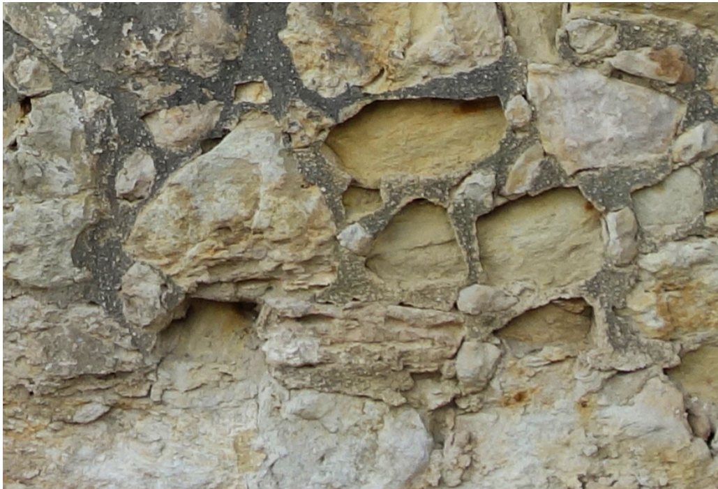
The depth of stone loss due to erosion varies from under 1 inch to 3 inches or more [wall between Long Barrack and Church].
