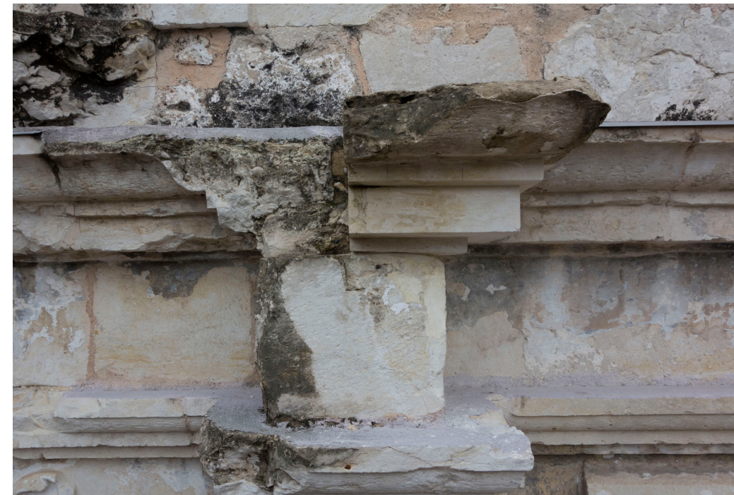
Severe loss of ornamentally carved material at the west facade of the Church.
