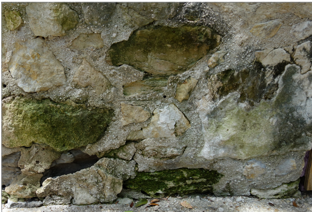
Biological growth that correlates with advanced deterioration at the base of the Long Barrack on the east elevation directly below the canals.
