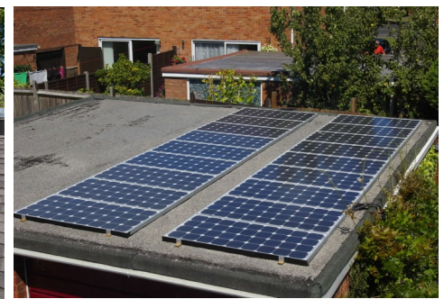
Appropriate mounting—slope and color
