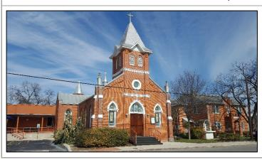
The Holy Redeemer Catholic Church is a brick masonry building of Neo-classical style with a center transept form. The sanctuary was built in 1927. The one-story sanctuary building features a centered steeple, double front door, standing seam metal roofing, arched stained glass windows and a large front gable. There is also a rose window and fixed windows with wood sashes. It retains a high level of its historic and architectural integrity. Meets criteria #1, 5, 8, 11, 13, and 15
