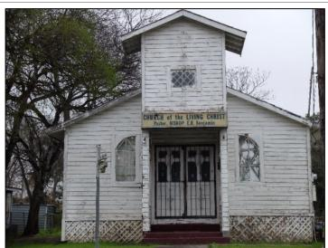
Single story wooden vernacular church with central tower with front gable and recessed entryway. Constructed c. 1922 and enlarged in 1924 for Immanuel Baptist Church. Windows along the nave have been replaced with narrow fixed windows. On the front façade, two windows flank the entry, and centered above the entry in the tower is a small rectangular window with diamond grid pattern. Meets criteria #1, 11, 13, and 15
