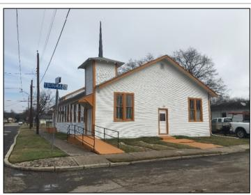
Wooden, front gabled with square tower at southwest corner with hipped roof and spire. Constructed in 1920, remodeled in 1958. 2 over 2 wood windows, eleven on west side and nine on east. Two story camelback on north end. South façade has single door in center, with two paired windows (2 over 2) on either side.
