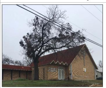
The Iglesia Met Dista Unida El Mesias is a brick masonry building of Mid-century Modern style. The construction date is estimated to be 1960. The onestory sanctuary building features a double front door, composition shingle roofing, and a large front gable with four small front gables in a chevron design. It retains a high level of its historic and architectural integrity.
