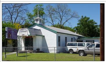
Constructed between 1966 and 1973 for Tried Stone Church. Stucco exterior, composition roof, portico with metal supports. Fixed metal windows. Rear wing with flat roof extends from rear of building to the east. Previously church building on north side of the same lot faced Lockhart. Meets criteria #1, 11, 13, and 15
