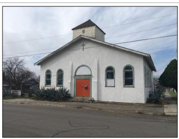
Built c. 1949, this single story stucco church building features one-over-one wood windows with half-moon transoms on the front, north, and south elevations. The front gabled roof has exposed rafter tails, and a square central tower rises above the front door which matches the windows with a large half-moon transom. A small side gabled wing protrudes from the rear of the south façade. This site was home to Greater Emmanuel AME from at least 1932 through 1985.
