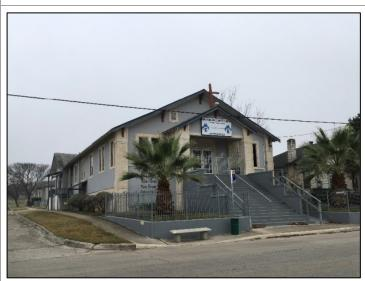
Originally founded as South Heights Church of Christ c. 1910, this single story structure has a full basement. The Craftsman style structure features exposed rafters, double front gables, and massive square porch supports. Modifications include paired picture windows, siding, and faux stone siding over the columns and basement. Church also owns single story Queen Anne house with wraparound porch and cutaway bay window facing Delmar.
