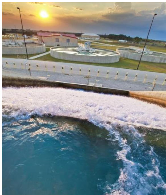
Figure 9-1: Raw water undergoes aeration, clarification and sand filtration at the SAWS H 2 Oaks Center treatment plant.
