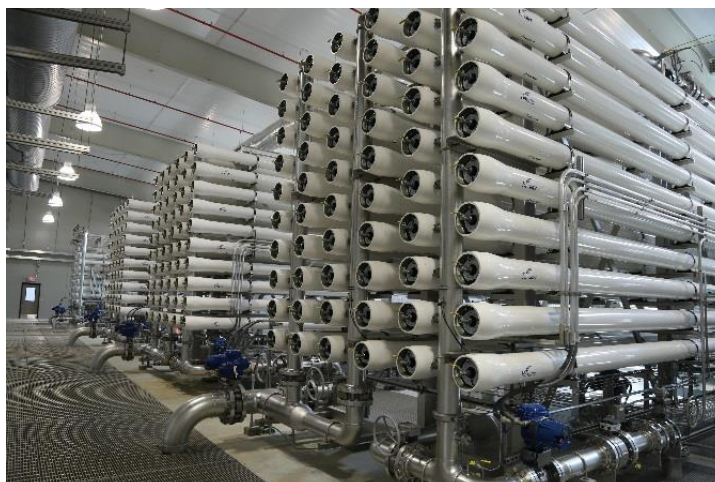
Figure 3-3: Racks of reverse osmosis membranes remove dissolved solids from brackish groundwater at the SAWS H 2 Oaks Center desalination plant in southern Bexar County.
