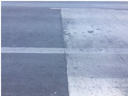
Intersection of Asphalt Pavement and Concrete bus stop
