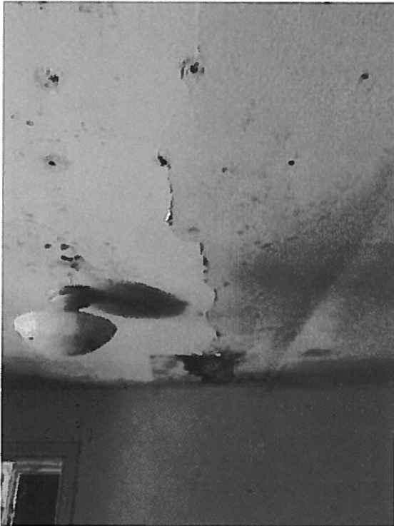
Photo 8: Cracking in Ceiling Sheathing
