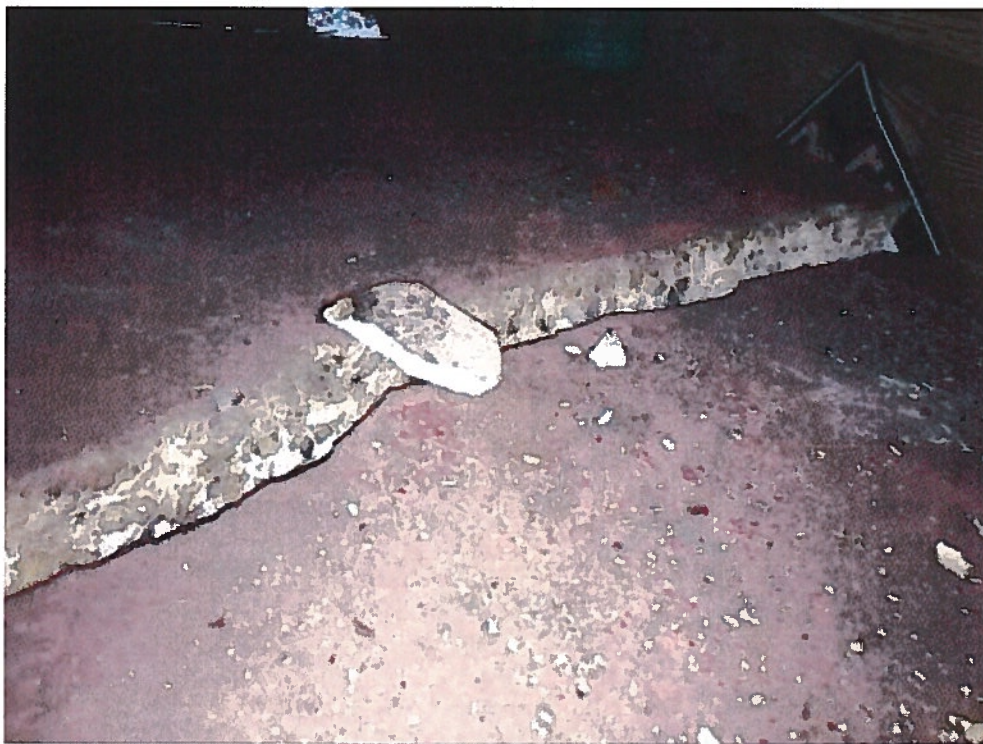
Photo 4: Concrete Slab Foundation Cracking and Movement
