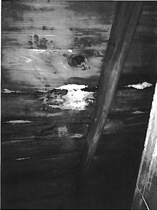
Photo 10: Signs of Fungus Infestation for Roof's Wooden Framing
