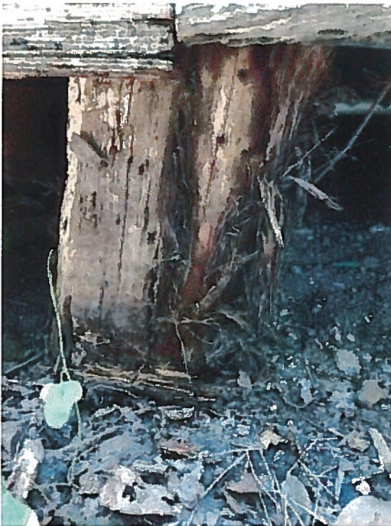
Photo 2: Timber Pile Foundation Loss of Section and Signs of Infestation
