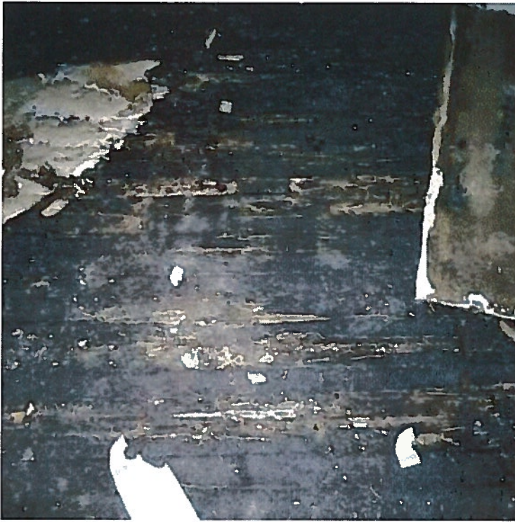
Photo 5: Typical Wood Flooring Deterioration
