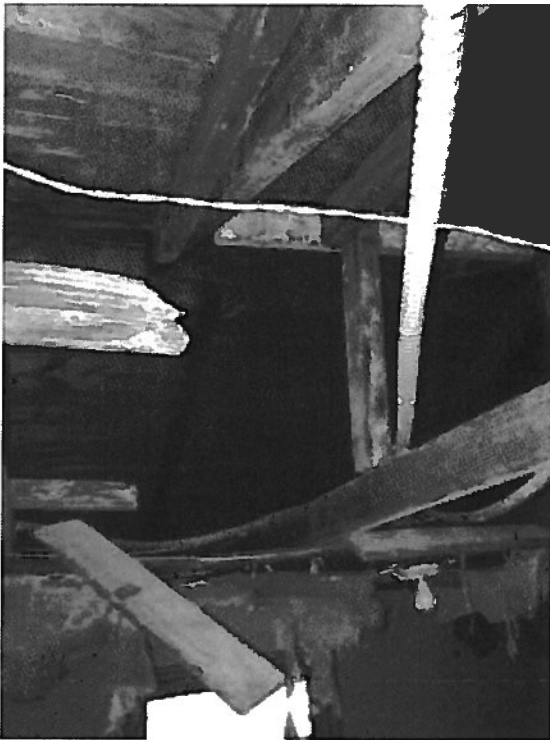
Photo 9: Collapsed Section of Wooden Roof Joists and Beams
