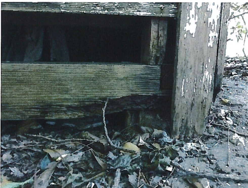
Photo 3: Wooden Beam Loss of Section and Bearing Area
