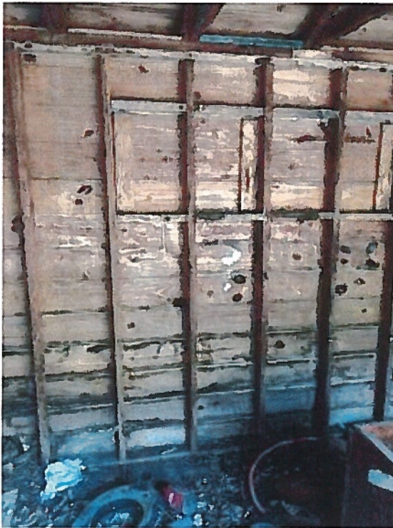
Photo 6: Wall Section with Multiple Signs of Fungus Infestation
