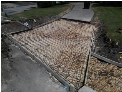
Above: demolished sidewalks in front of residential properties on La Manda Street near Scales Street, in preparation for precast sidewalk construction Above: forms installed for a driveway, transitions, and a corner with grading—elements that are not conducive to precast construction
