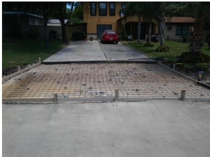
Above: demolished sidewalks in front of residential properties on La Manda Street near Scales Street, in preparation for precast sidewalk construction Above: forms installed for a driveway, transitions, and a corner with grading—elements that are not conducive to precast construction
