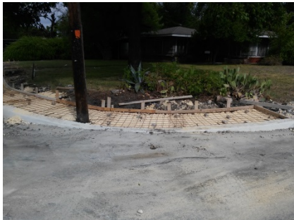
Above: demolished sidewalks in front of residential properties on La Manda Street near Scales Street, in preparation for precast sidewalk construction Above: forms installed for a driveway, transitions, and a corner with grading—elements that are not conducive to precast construction
