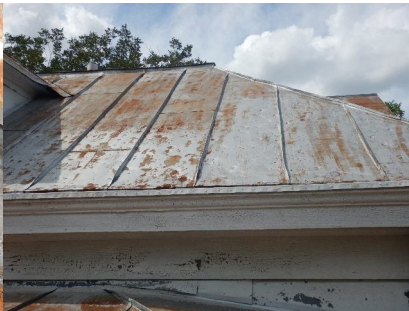
Rust and dents to metal roofing
