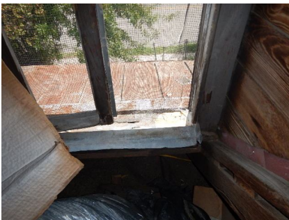
Broken window in attic
