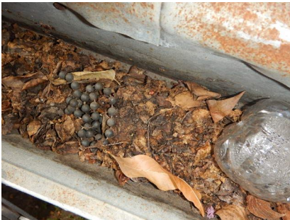
Debris in gutters
