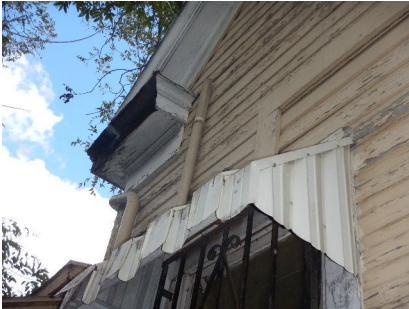
Vent stack does not pass roof line
