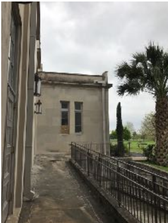
6. View east along south exterior wall showing downspouts discharge directly on concrete walkway that slopes toward building. Work intended to provide positive drainage through installation of underground extensions to downspout. Concrete walk to be removed and replaced.
