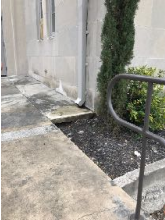
5. Condition at the area where downspout meets the walkway. Negative slope towards the building to be corrected and underground drainage to be installed. Concrete walk to be replaced.
