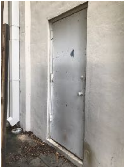
8. Detail showing downspout at stage door. downspouts discharge directly on concrete walkway that slopes toward building. Work intended to provide positive drainage through installation of underground extensions to downspout. Concrete walk to be removed and replaced.
