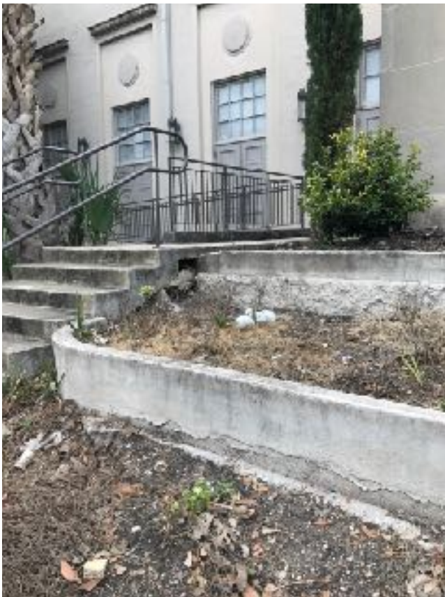
4. South elevation detail showing the erosion at the walkway and stairs, to be replaced.
