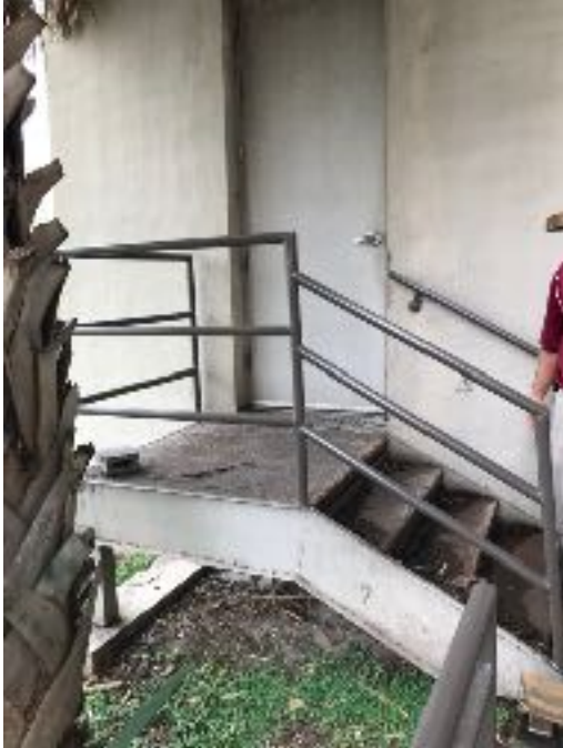
7. Exterior steel stairs located at west end of Southern exterior wall to be replaced with concrete steps to match existing.
