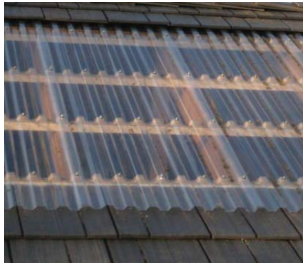
CORRUGATED POLYCARBONATE ROOF COLOR: TO MATCH EXISTING
