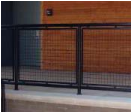
FENCE TYPE 1 DESCRIPTION: STEEL ANGLED WITH 2X2 METAL MESH WELDED TOGETHER PAINTED: BRONZE (ACCESS GATES SIMILAR)
