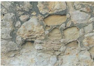
The depth of stone loss due to erosion varies from under 1 inch to 3 inches or more [wall between Long Barrack and Church].
