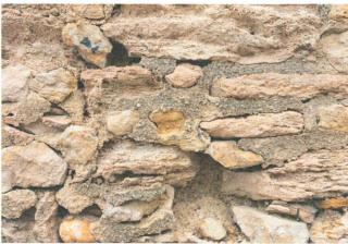
Severe material loss in the zone of rising damp.
