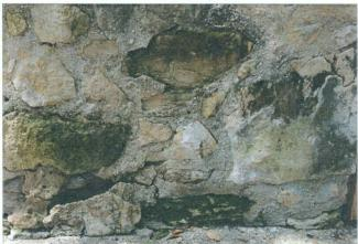
Biological growth that correlates with advanced deterioration at the base of the Long Barrack on the east elevation directly below the canales.
