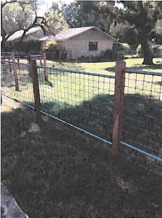
Fence: Cattle Panel & posts; Horizontal wood slats (6ft high)
