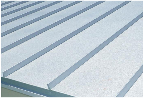
STANDING SEAM METAL ROOF COLOR: GALVALUM (PANELS - 18"-21" WIDE, SEAMS 1"-2" IN HEIGHT, CRIMPED RIDGE SEAM)
