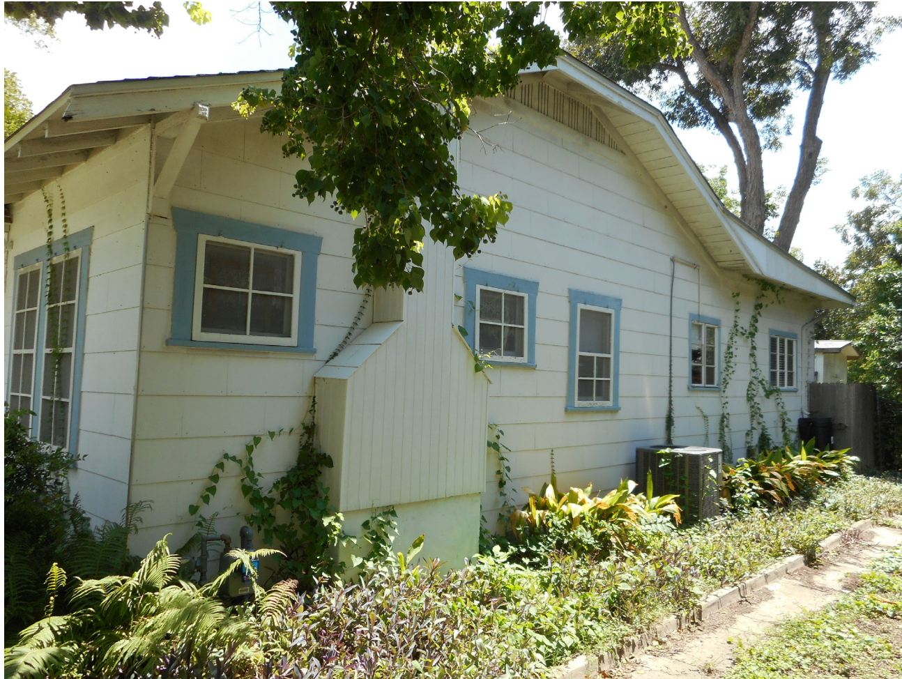
WEST FACADE: Areas of work include re-cladding the exterior faces of the fireplace and chimney with brick. The original brick had deteriorated and was replaced with painted siding in a previous renovation.
