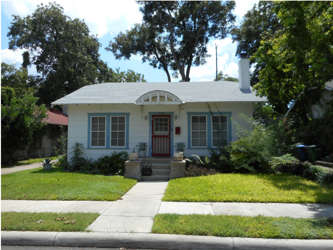
STREET VIEW / NORTH FACADE: Areas of work include replacing the brick and concrete stoop (not original to the historic structure) with a wood porch. Work also includes re-cladding the exterior faces of the fireplace and chimney with brick.
