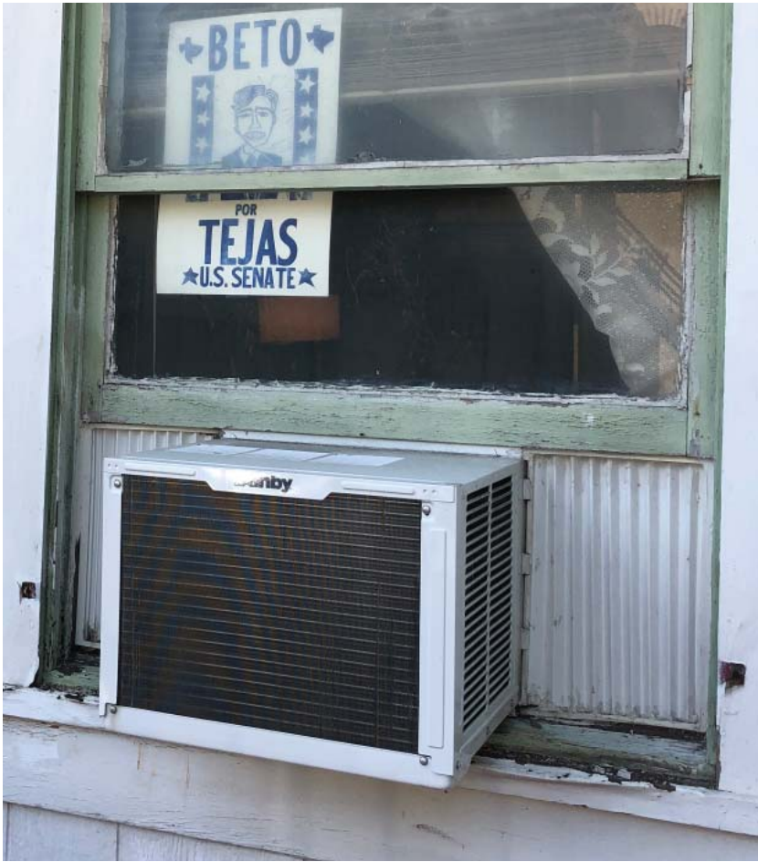
Window sill rot at existing window. Window is proposed to be replaced.
