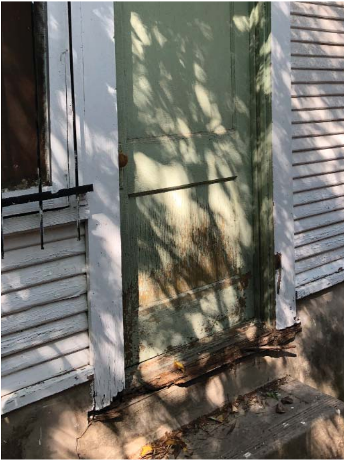
Door rot at an east elevation exterior door. Door and concrete steps are proposed to be removed given they were not part of the original design intent.
