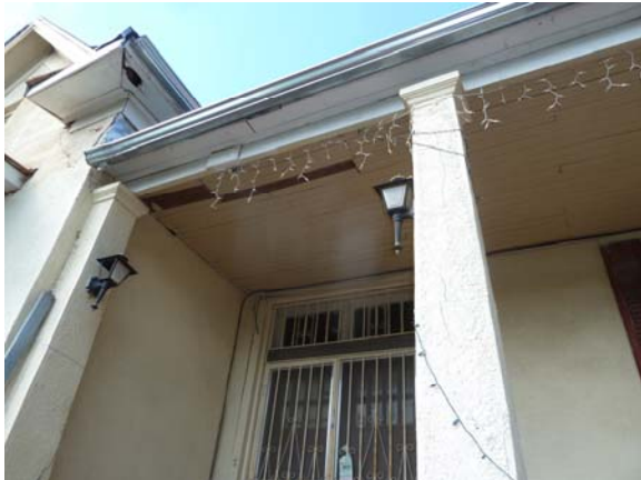
Wood rot of trim materials and possible rot of underlying structural members especially on the “Addition”.
