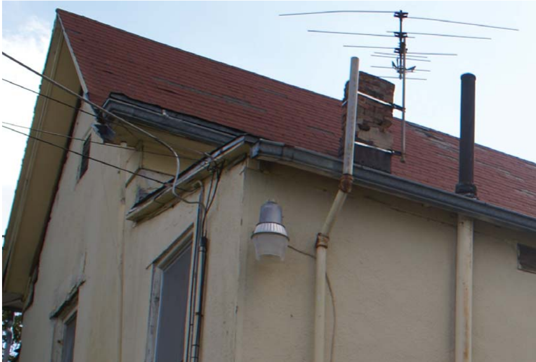
ABANDONED CHIMNEY TO BE DISASSEMBLED AND ENCAPSULATED BELOW ROOFLINE
