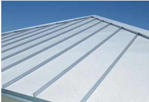
GALVANIZED STANDING SEAM METAL ROOF
