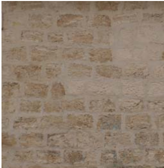
REPOINTED AND STABILIZED CALICHE BLOCK, EXPOSED
