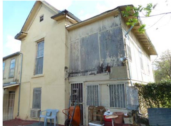
Wood rot of trim materials and possible rot of underlying structural members especially on the “Addition”.
