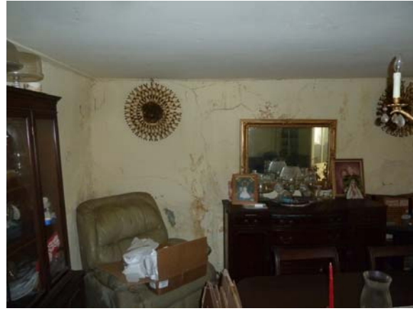
Interior first floor wall showing moisture.
