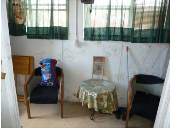
Efflorescence from exterior moisture, front wall.
