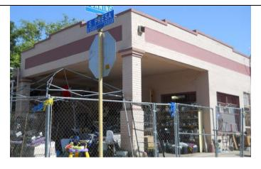
This Classical Revival brick structure has massive square columns with tapered brick pedestals and cast stone capitals and a flat roof with stepped parapet. The canopy extends from the office which shares the parapet-roofline. Insets for signage are still visible on the side and front of the canopy. Original windows topped with narrow transoms remain intact.
