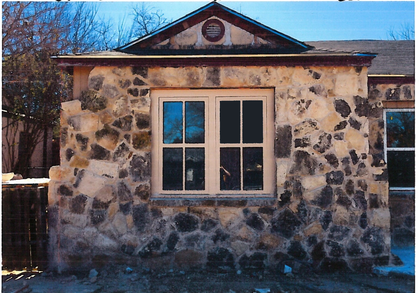
STONE INSTALLED AROUND FRONT LEFT WINDOW
