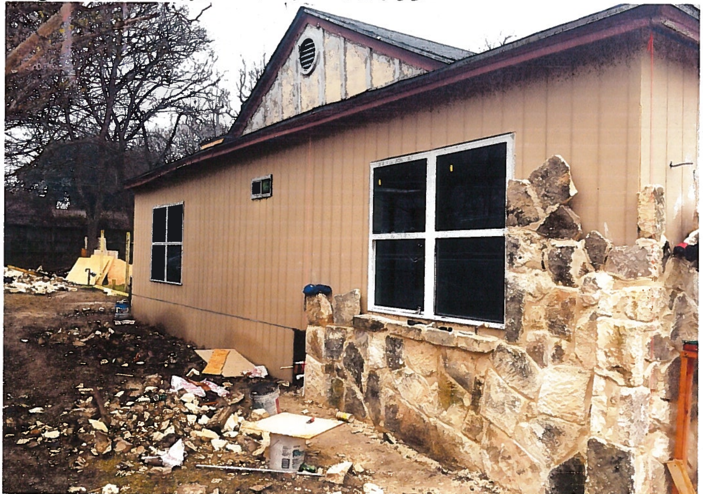
STONE INSTALLATION IN PROGRESS
