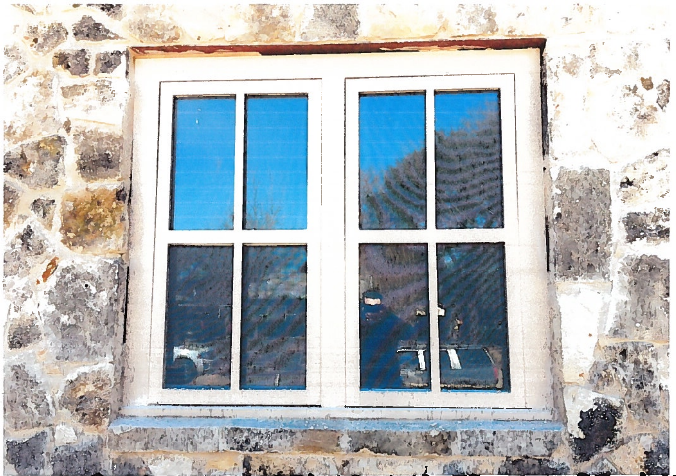
STONE INSTALLED AROUND FRONT LEFT WINDOW
