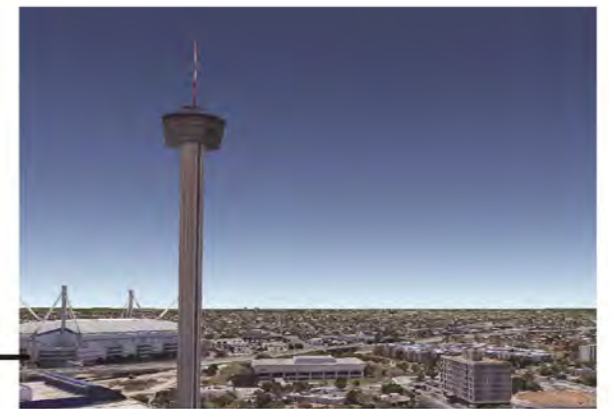
Southeast view out onto Hemisfair park and the Tower of the Americas beyond
