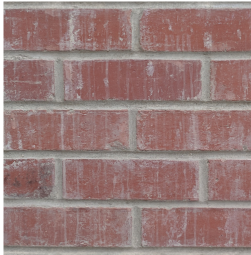
EXISTING BRICK PAINT REMOVED
