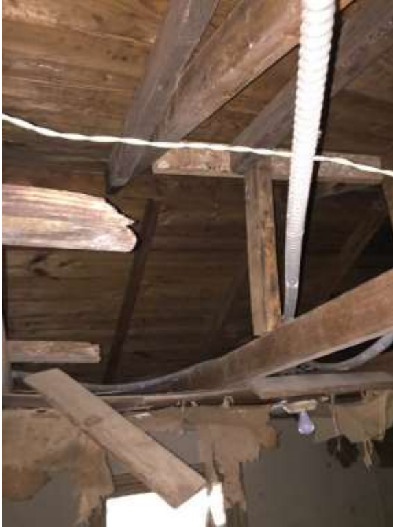
Photograph of damaged wooden roof framing with a white corrugated pipe running through it.
