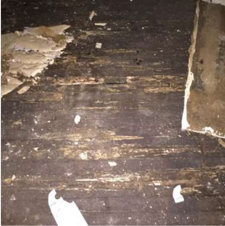
Figure 5: Close-up of damaged wooden floor joists.
