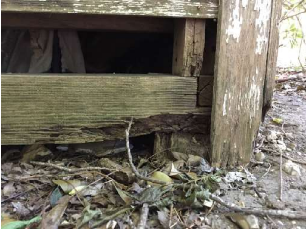
Figure 4: Severe rot and decay in the wooden joists and support posts of the structure.
