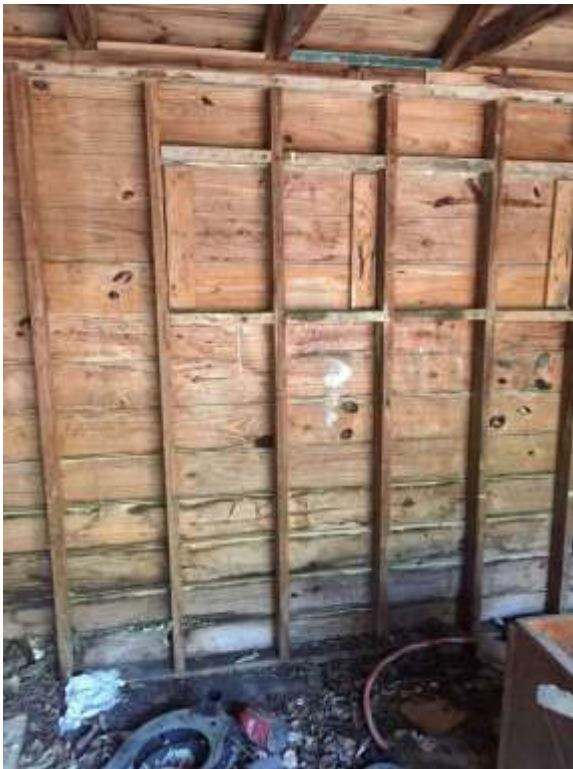
Figure 6: View of wooden wall structure showing vertical studs and horizontal planks.
