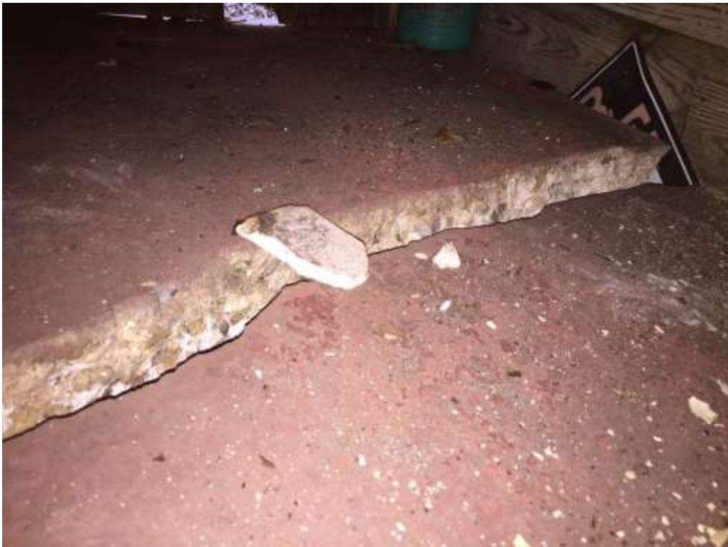
Figure 4: Cross-section of the concrete foundation showing severe deterioration and hollowing.
