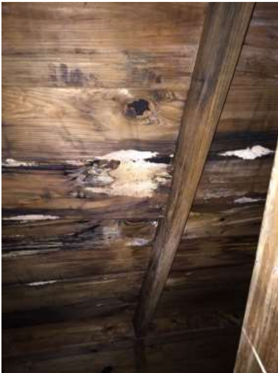
Close-up photograph of a wooden beam showing signs of fungus infestation for roof's wooden framing
