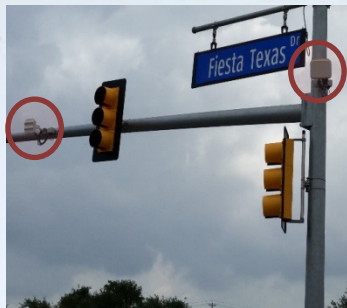
Steel Mast Arms & Vehicle Detection
